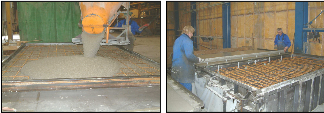
Figure 2.3 Example of a simple horizontal casting (wall element) in the precast industry. Filling and finishing are shown to the left and right, respectively (Rottig 2003).
