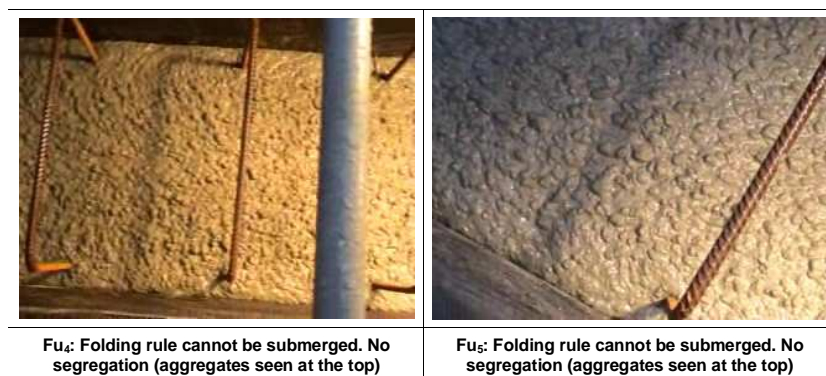
Figure 7.57 Photos of the top surface after casting in form filling applications Fu_4 and Fu_5 . A folding rule has been used to indicate the distance between the top surface and the coarse aggregate.
