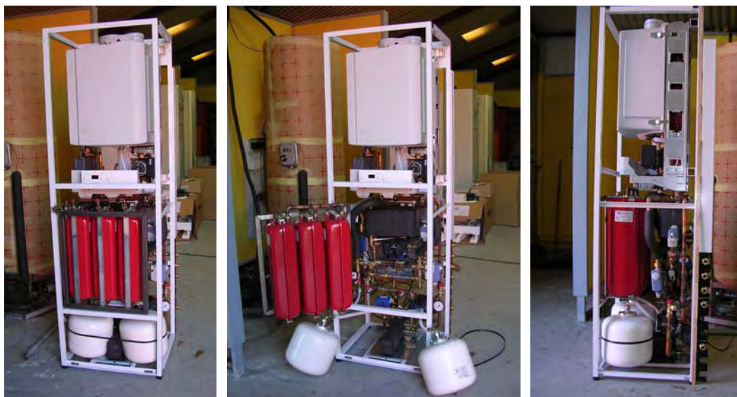
Fig. 3–7 Technical Unit, ready for installation in the demonstration house
