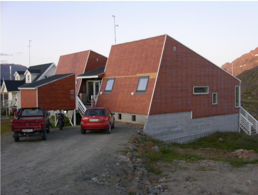
Figure 31 Low-energy house and fixing of windows in inclined wall
