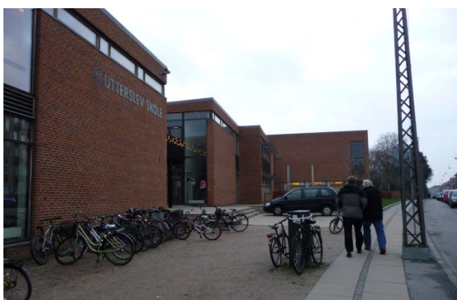
View of the administration building from the street
