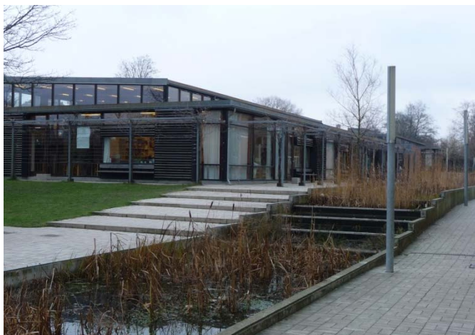
School building 1 viewed from channel area
