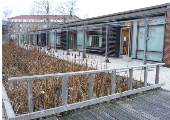
School building 3 viewed from channel area
