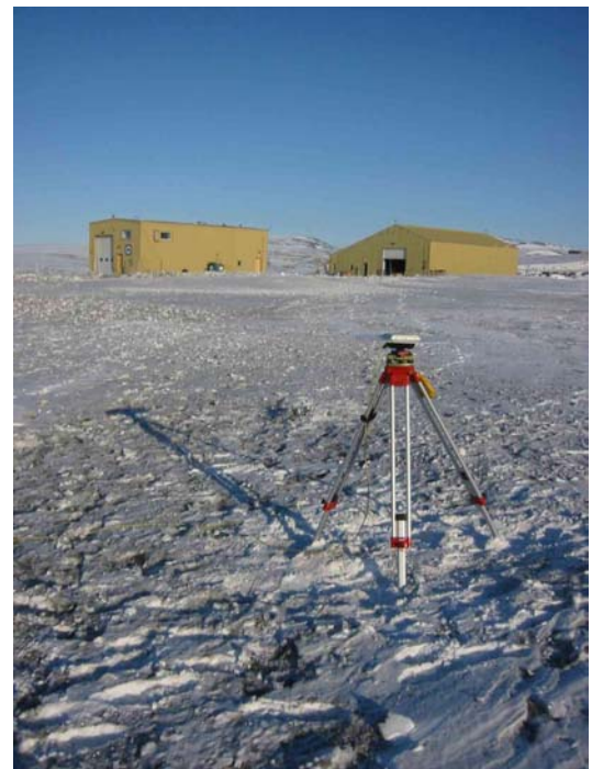
Fig. 5. The GPS references in Alert, YLT1 in front, YLT2 on top of the leftmost building
