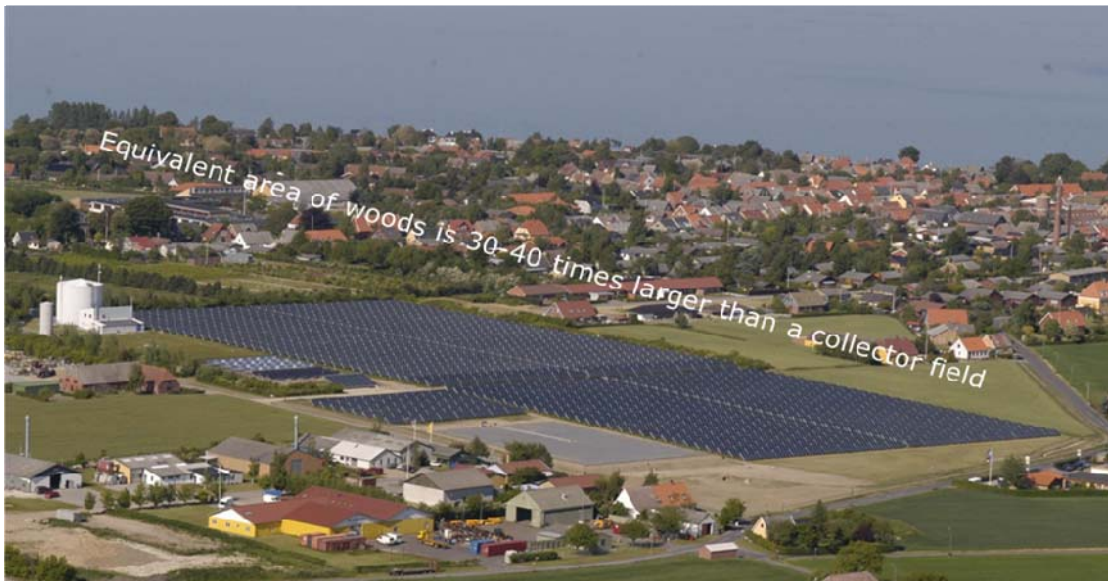
Figure 4. Marstal Solar Collector field connected to the local cogeneration power station and district heating network.
