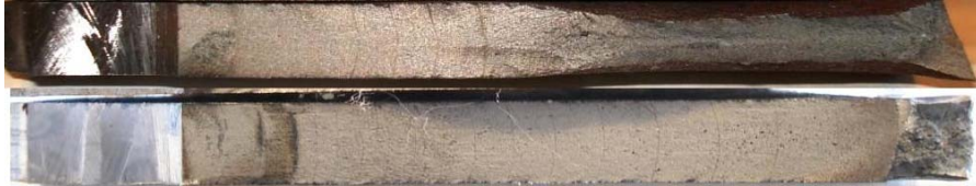
Figure 4. Cross section of a reference and a typical strengthened specimen after failure.
