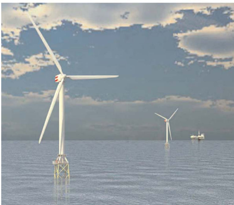
Figure 5.1: The Beatrice wind farm consisting of two 5 MW wind turbines in 42 m deep water. The wind farm is connected to an existing oil production facility. Source www.beatricewind.co.uk
