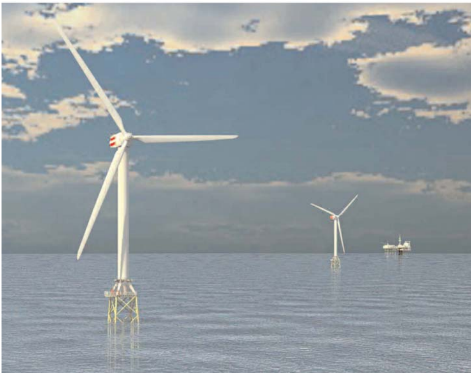
Figure 5.1: The Beatrice wind farm consisting of two 5 MW wind turbines in 42 m deep water. The wind farm is connected to an existing oil production facility. Source www.beatricewind.co.uk
