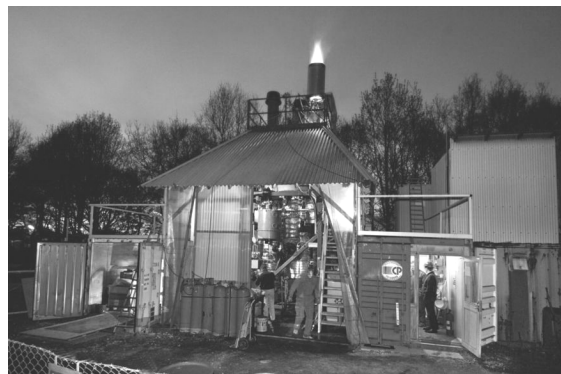
Figure 2: 500 kW LT-CFB plant at DTU
