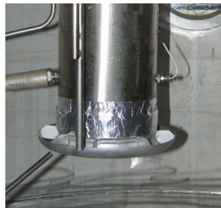
Figure 2. Collar of the blowdown pipe.
