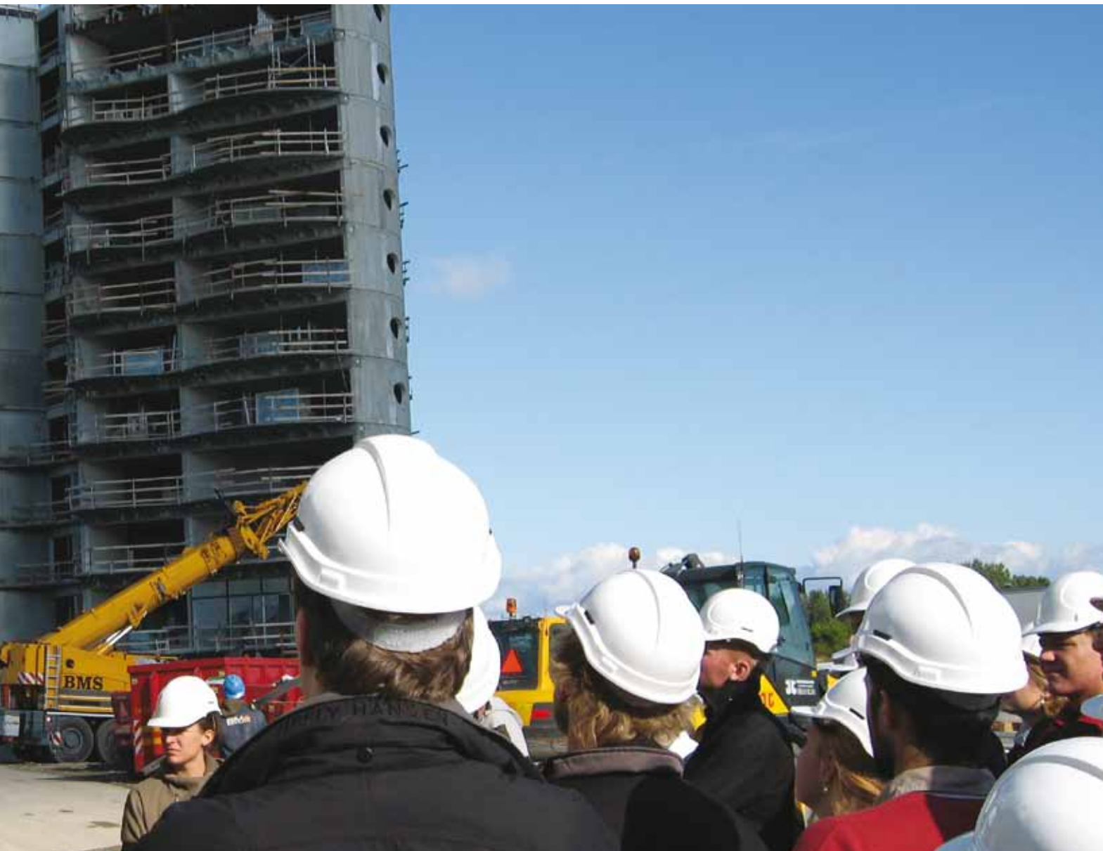
Introduction to the construction site, safety and the building process with all its challenges in high-rise structures. Photo: Per Goltermann
