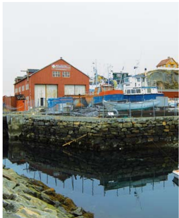
Nutaaliorfik – the Greenland Innovation Centre is situated in the old shipyard in the Sisimiut harbour.
