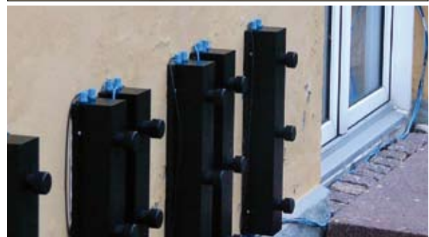
The electrochemical method for salt removal is not only applicable for church vaults. It can also be used for salt extraction from infected masonry of normal houses and a pilot plant for such treatment is seen here
