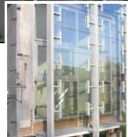
Fig. 1 The solar shading system with the lamellas in daylight redirecting position.
