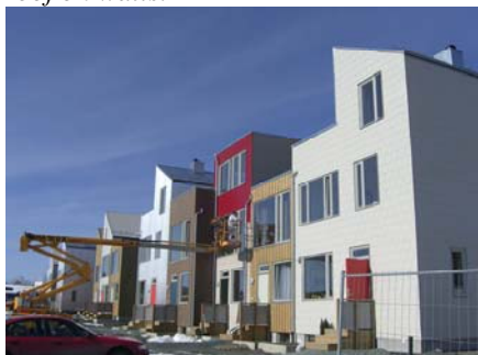
Fig. 5 Modern dwellings built of massive timber element
