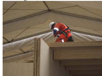
Fig. 4 It is recommended to raise massive timber constructions using Weather Protection Systems
