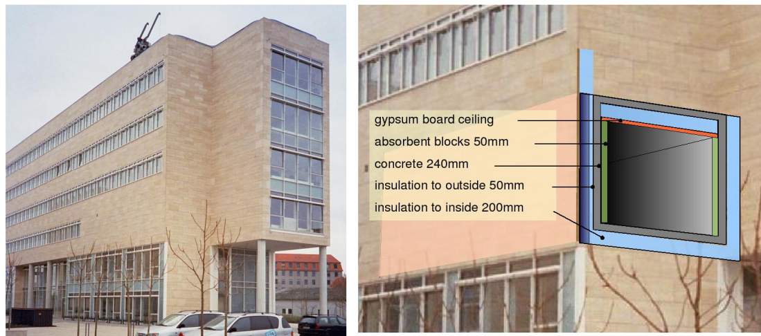
FIG. 1: The archive of the Arnemaganaean Institute of Copenhagen University is concealed behind the windowless area of the building (left). The archive, sectioned in the right hand picture, is insulated against both the internal and the outdoor temperature, so that its temperature is always about half way between the constant 22°C of the building and the variable outdoor temperature.
