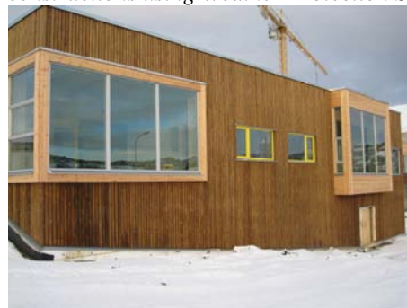
Fig. 6 Part of a new school being built in massive timber
