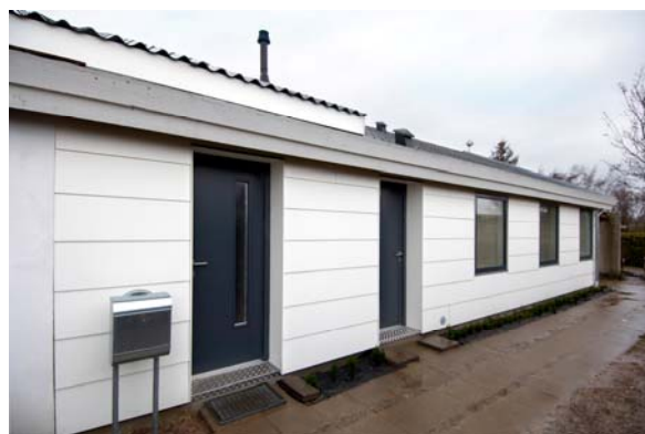
Fig. 3. House façade to the south after the renovation.
