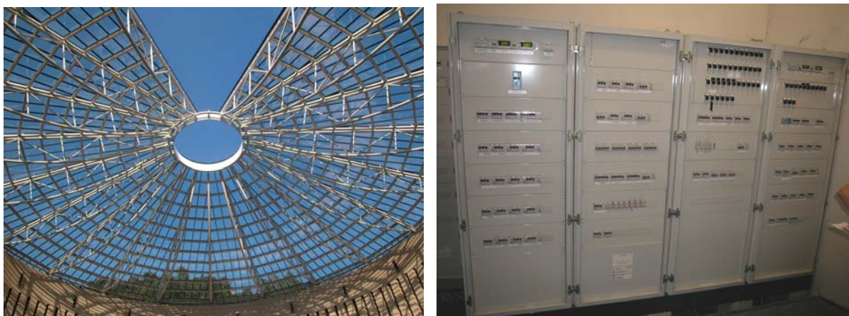
FIG. 2: Glass couple on the museum square (left side); electric cabinet for the manual centralized control of the previous system.
