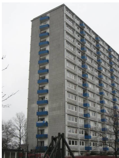
FIG. 2: The gables of the 14 storey houses consist of relatively uninterrupted concrete sandwich panels.
