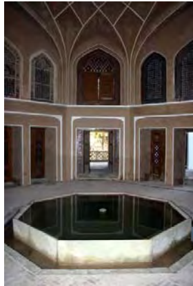
Fig.4 Room of under wind tower with small pool to moisture of weather
