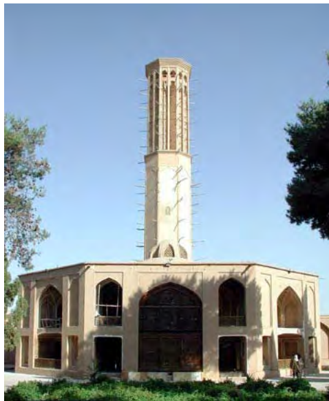
Fig.1 Wind tower of Doulat-Abad garden of Yazd with its altitude is 33 meters and 80 centimeter. It is highest wind tower in Iran. It has built in 1750. This wind tower has octagon plan. It can receive wind from eight directions and conduct it inside of room.
