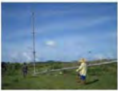
Raising-up the tower
