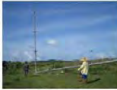
Raising-up the tower
