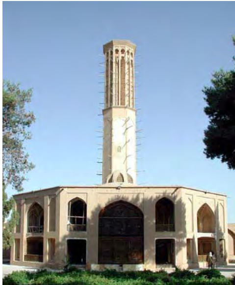
Fig.1 Wind tower of Doulat-Abad garden of Yazd with its altitude is 33 meters and 80 centimeter. It is highest wind tower in Iran. It has built in 1750. This wind tower has octagon plan. It can receive wind from eight directions and conduct it inside of room.
