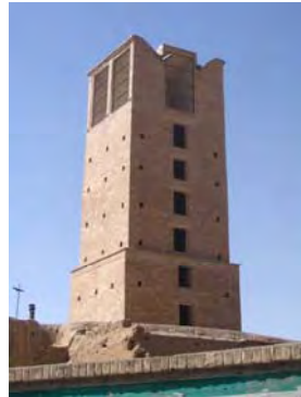
Fig.7 Rajabi wind tower is highest wind tower in Semnan and its altitude is
