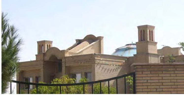
Fig.2 a new building equipped in wind tower in Semnan
