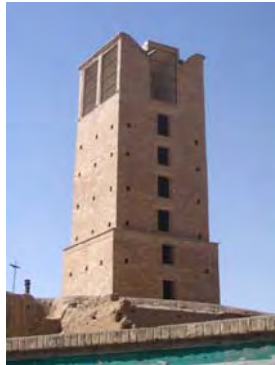
Fig.7 Rajabi wind tower is highest wind tower in Semnan and its altitude is
