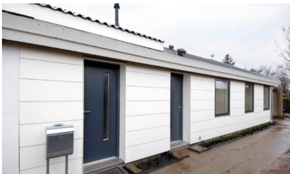
Figure 10: A typical Danish single-family house from the 1960s or 1970s (Næstved). It was retrofitted in 2006 to roughly the energy performance of a new Danish single-family house.
