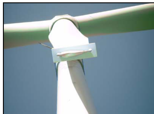
Figure 6: The five hole pitot tube mounted on the leading edge of the blade. (The plate mounted on the blade is used for measurement of the angle of the pitot tube relative to the tip pitch).
