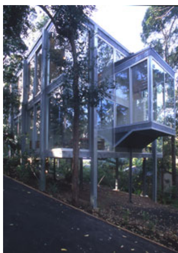
Fig 4: Malcolm Carver's Beach House from 2005 in New South Wales, Australia uses self-cleaning glass.
