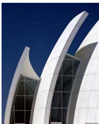
Fig 1: Richard Meier's Jubilee Church using nano coating on concrete panels
