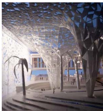
Fig 5: Henning Larsens Tegnestue’s Institute for Diplomatic Studies, Riyadh. Speculative project exploring complex glass surface that could use nano-glass.
