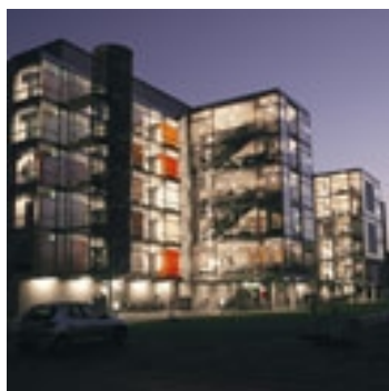
Fig 3: Lundgaard og Tranberg's Industri Kollegiet in Copenhagen uses a TCnano's gel compound for floor sealing.
