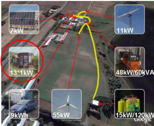
Figure 2. Components in SYSLAB
