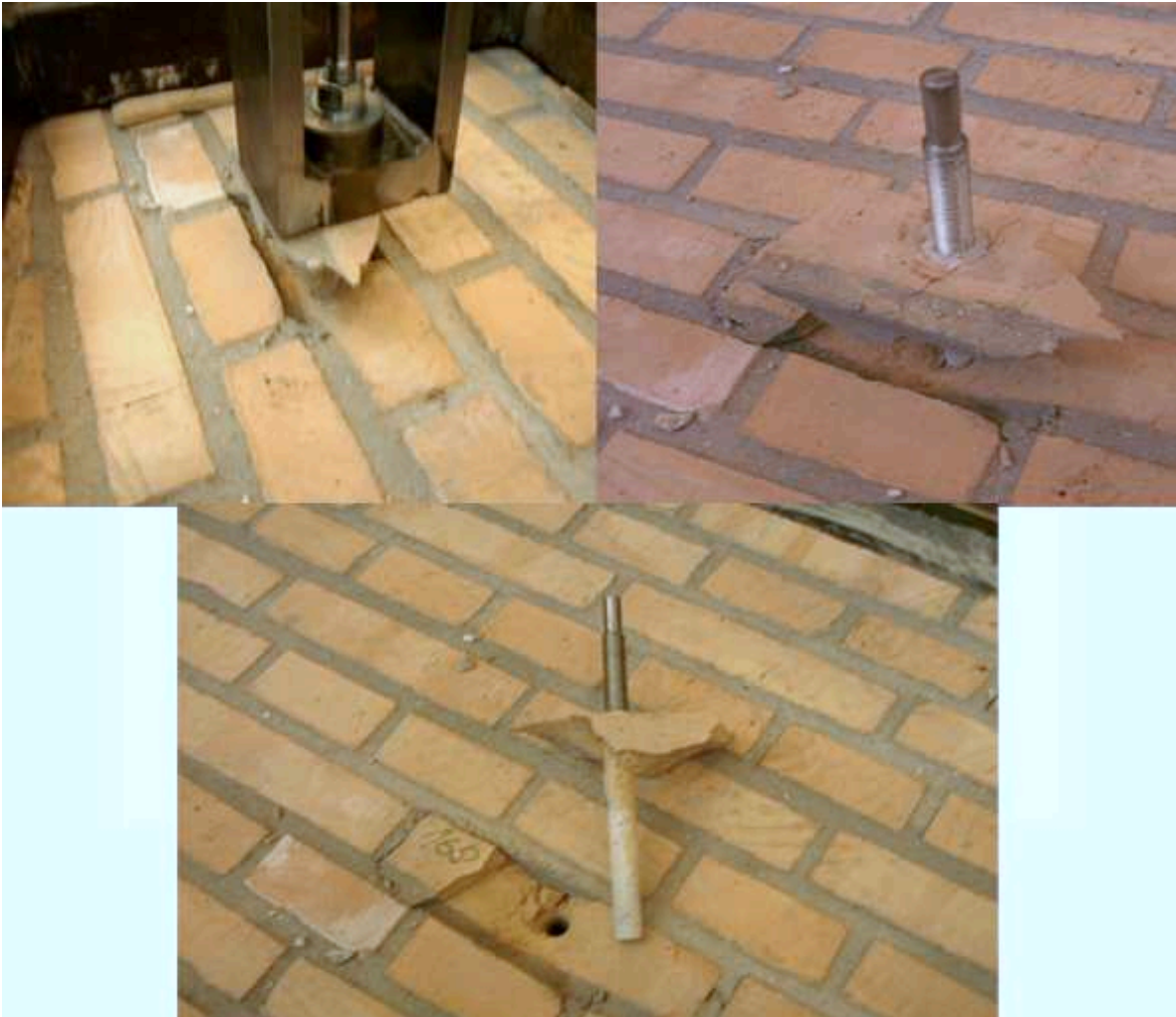
Figure A.37: The failure mode observed
