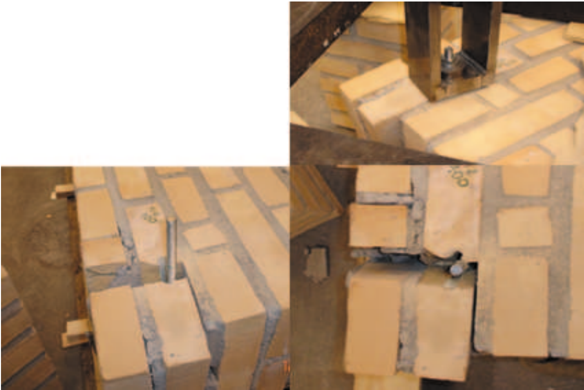
Figure A.109: The failure mode observed
