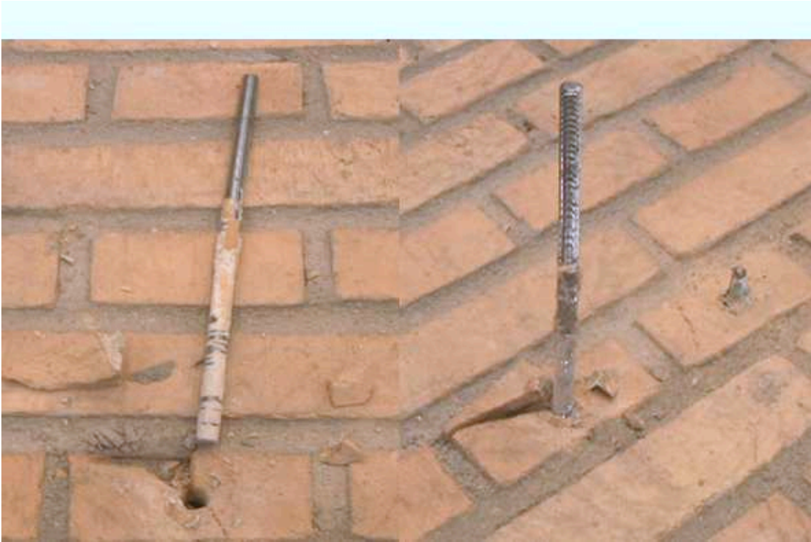
Figure A.65: The failure mode observed
