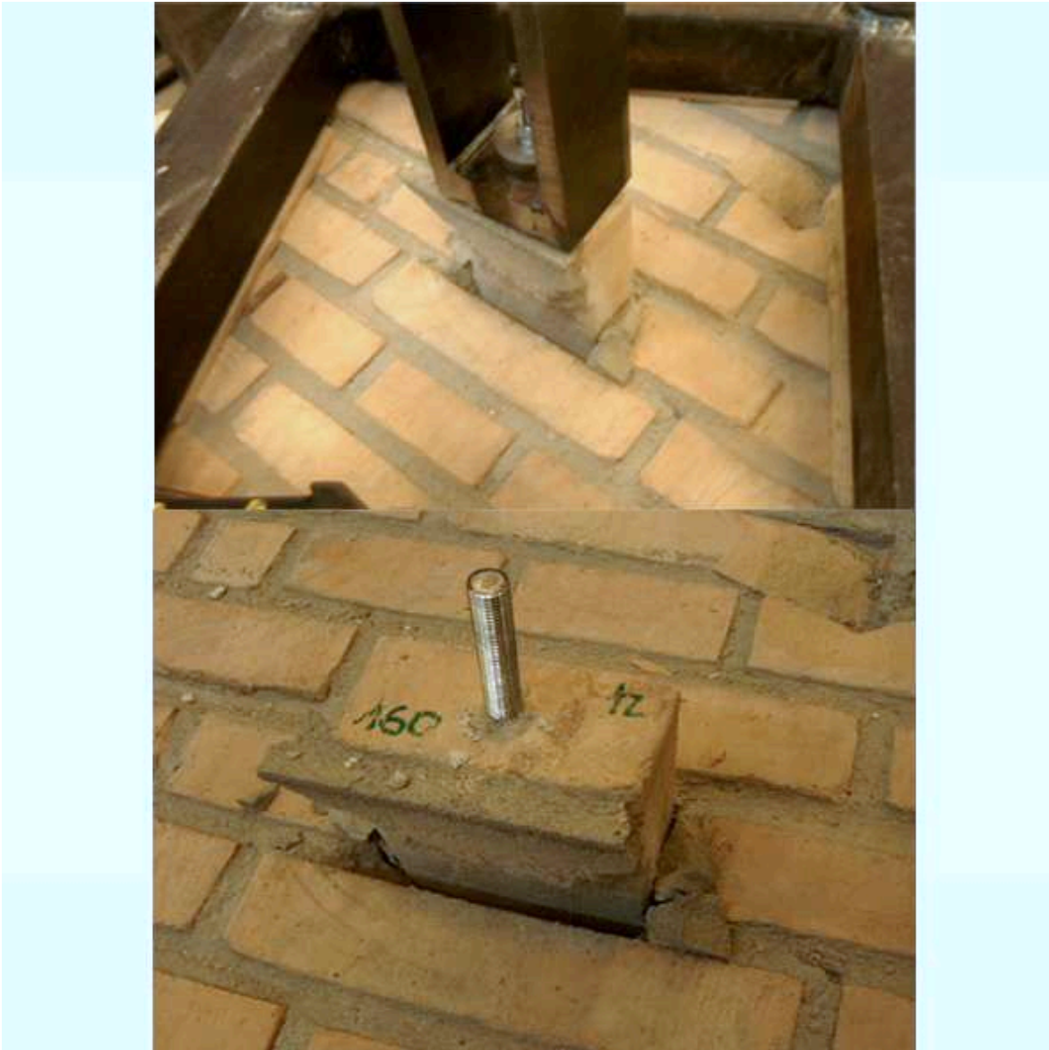
Figure A.75: The failure mode observed
