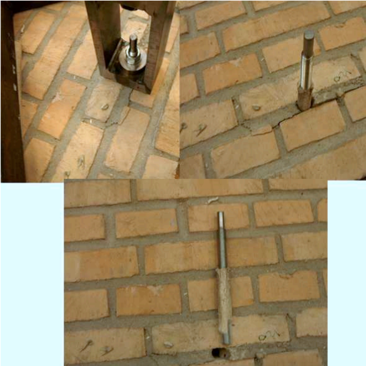
Figure A.103: The failure mode observed
