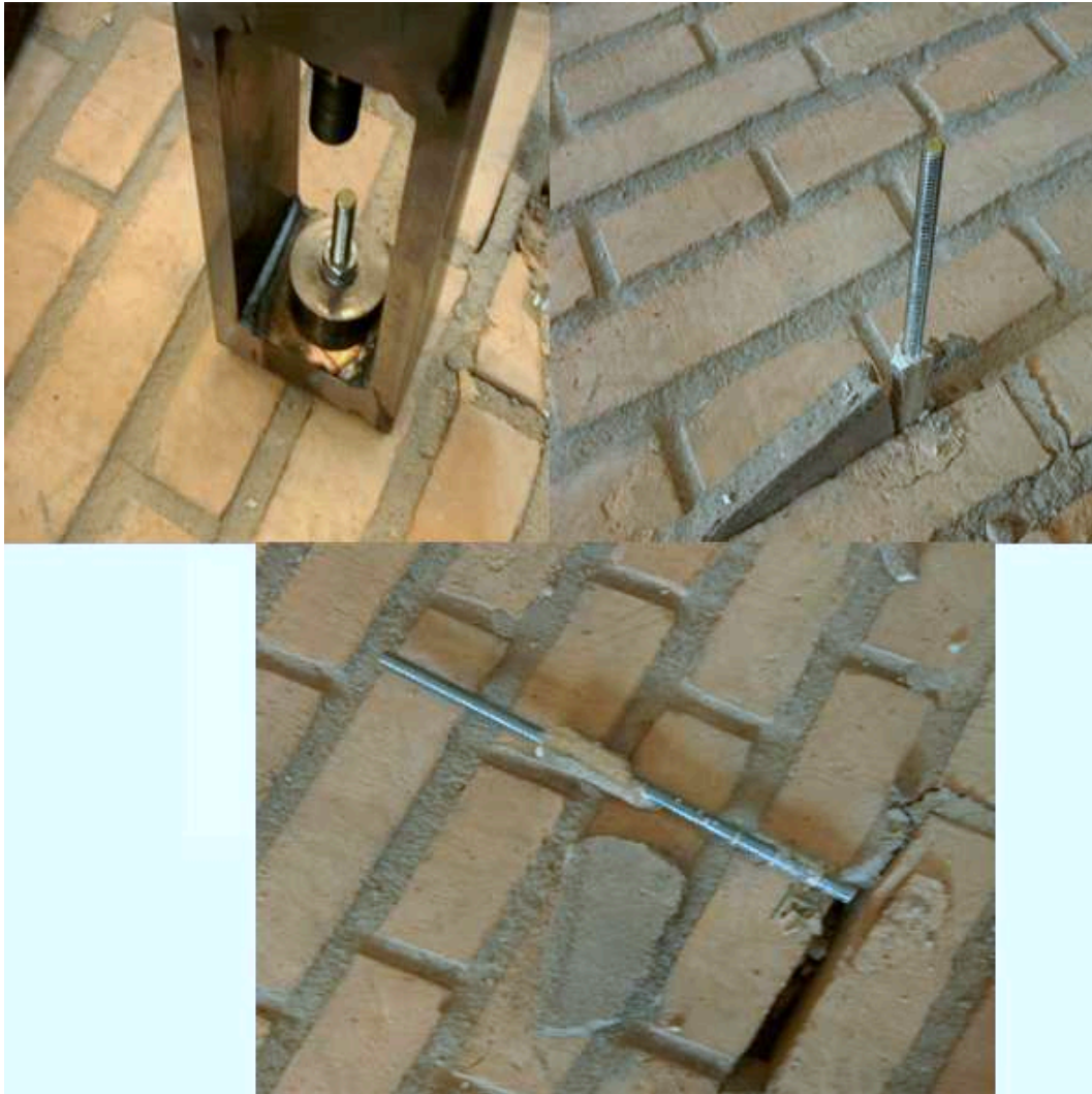
Figure A.91: The failure mode observed
