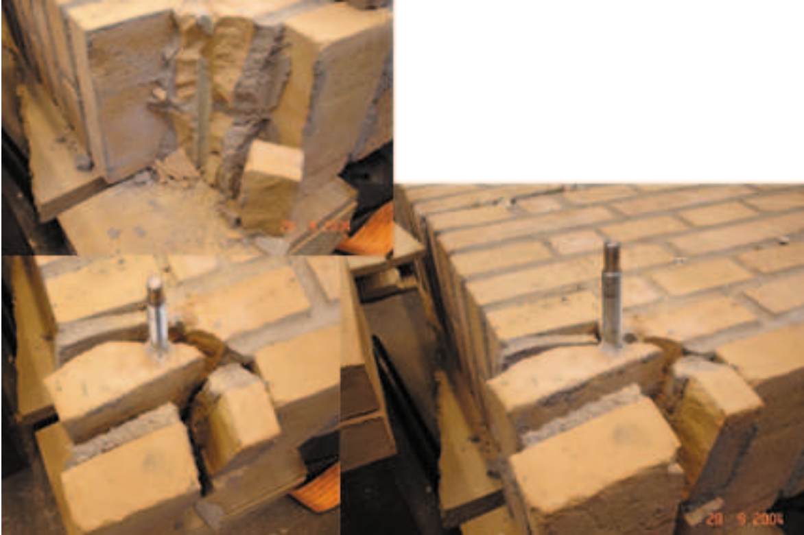
Figure A.117: The failure mode observed
