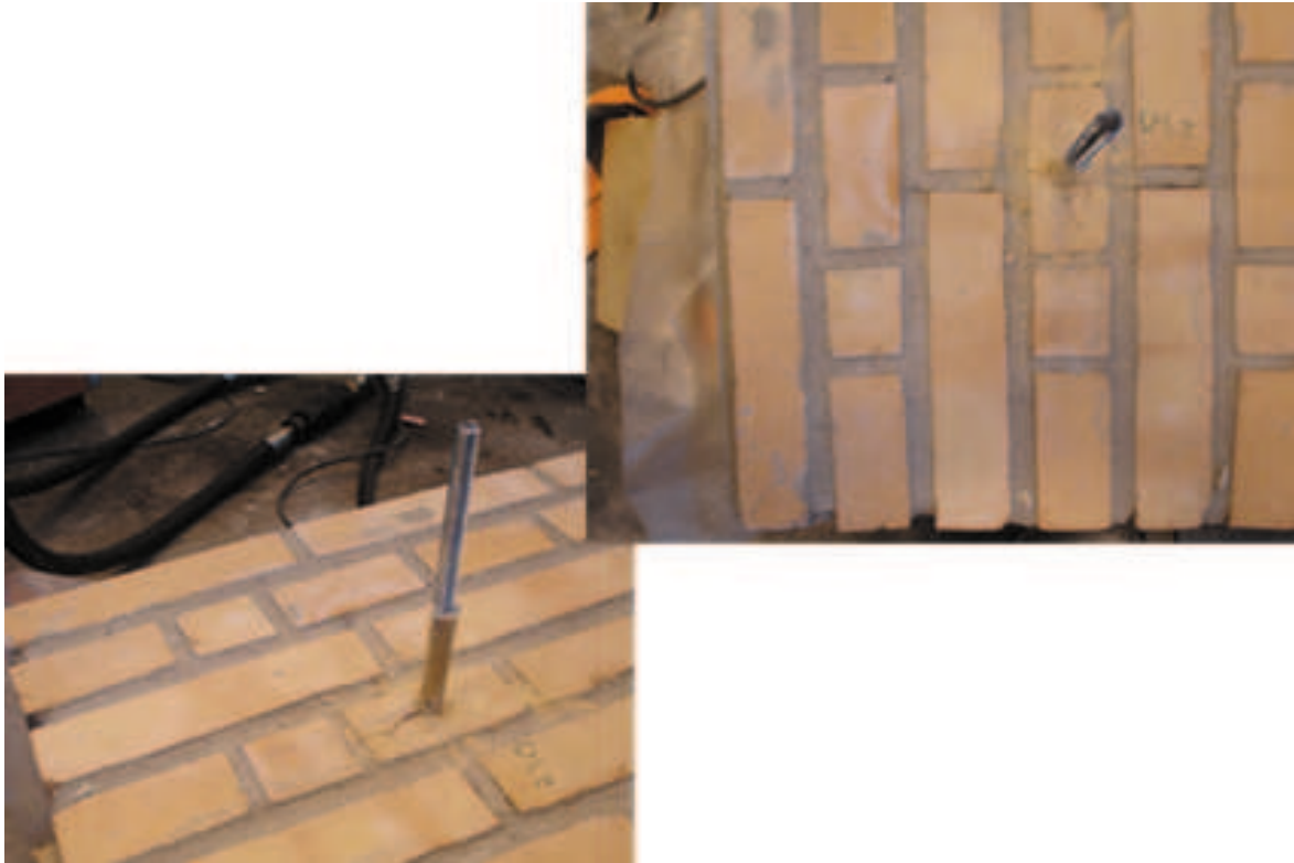
Figure A.113: The failure mode observed
