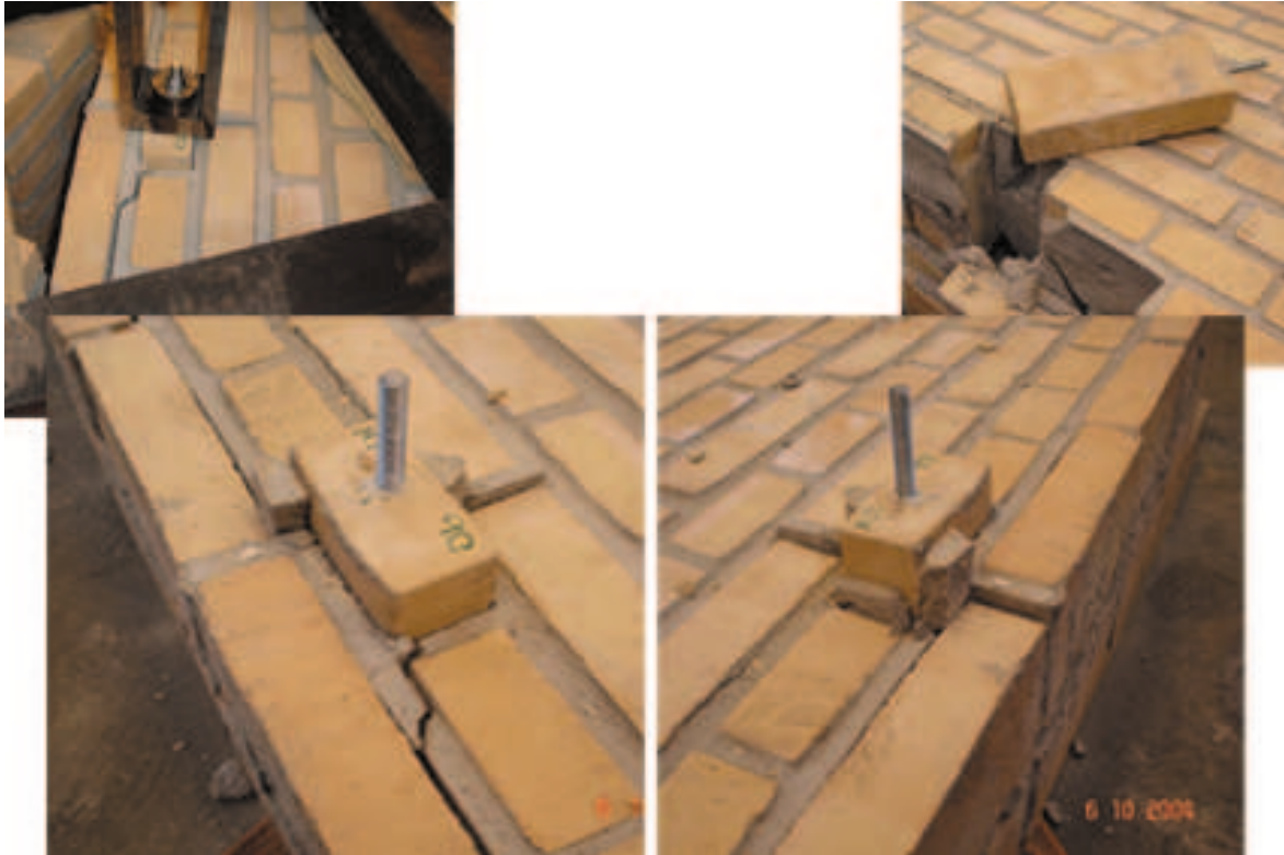
Figure A.139: The failure mode observed
