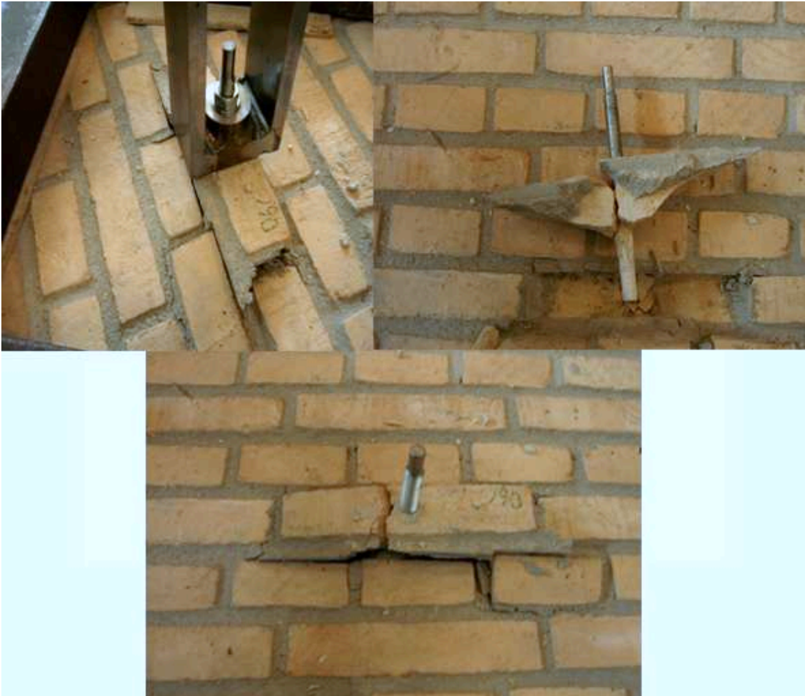
Figure A.35: The failure mode observed
