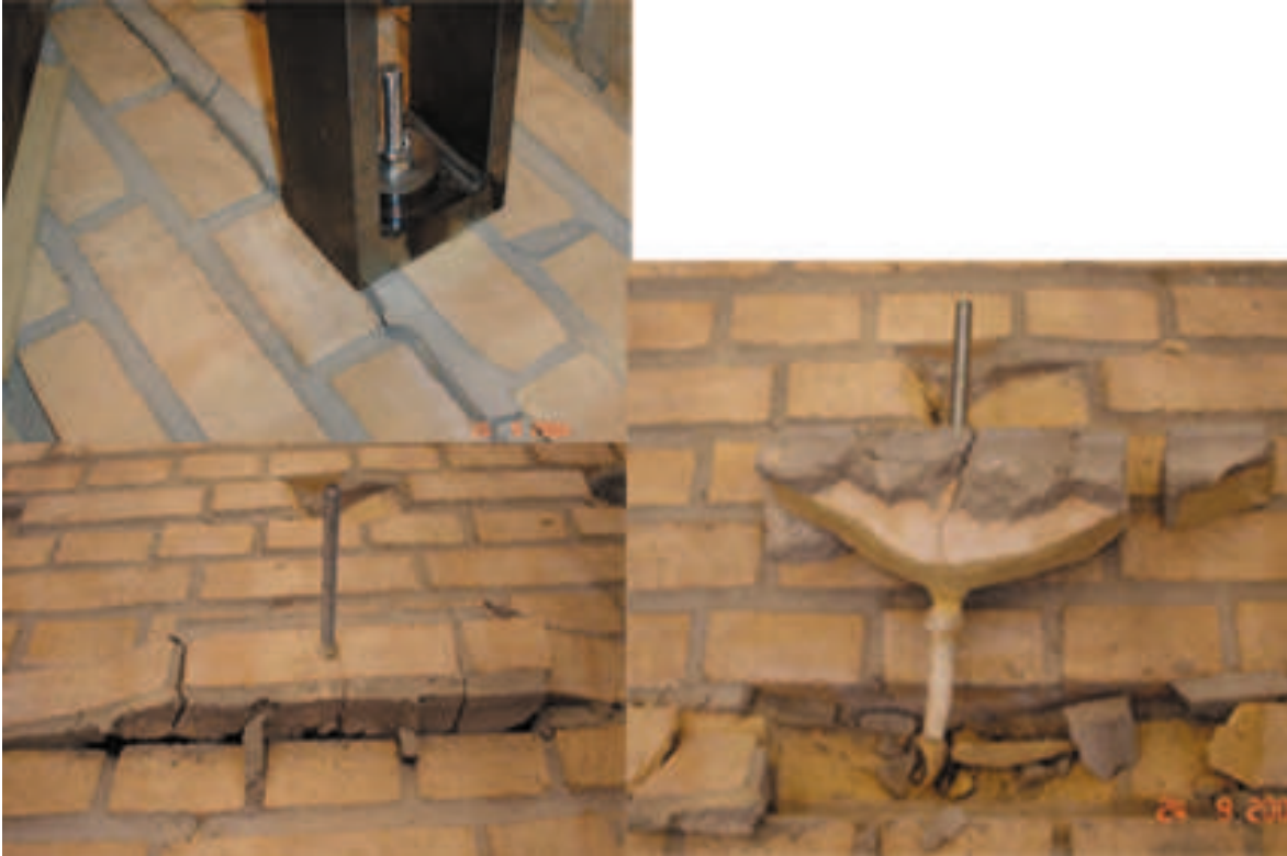
Figure A.5: The failure mode observed
