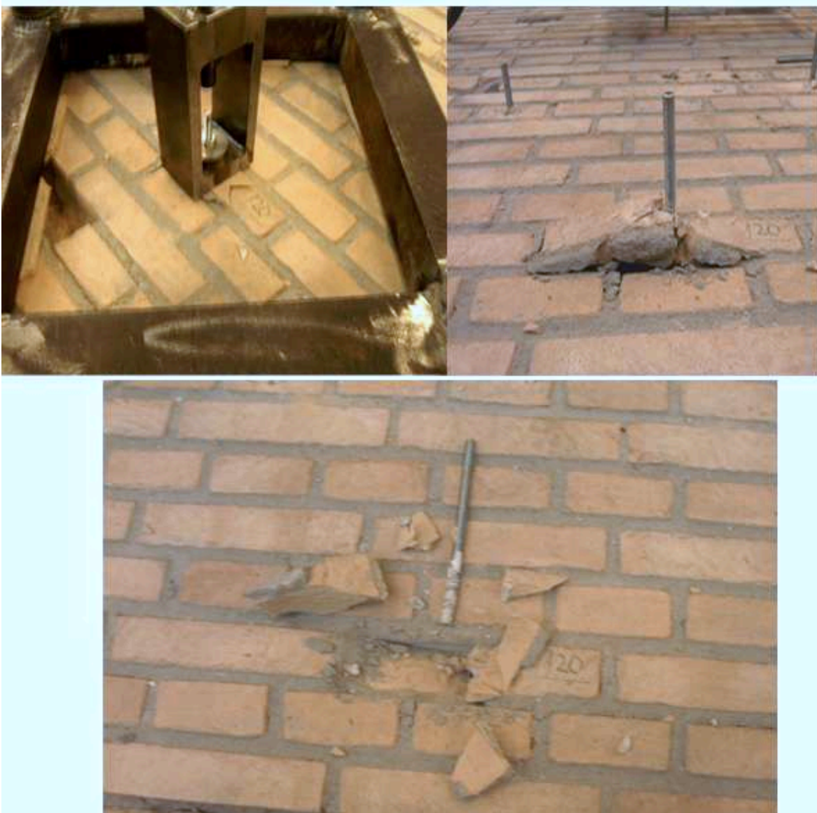
Figure A.17: The failure mode observed
