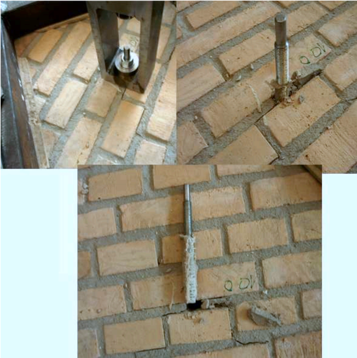
Figure A.101: The failure mode observed
