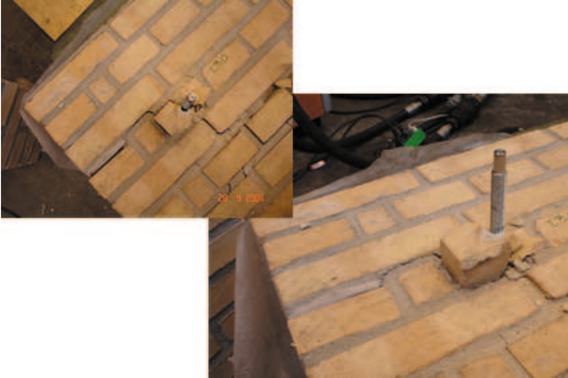
Figure A.123: The failure mode observed
