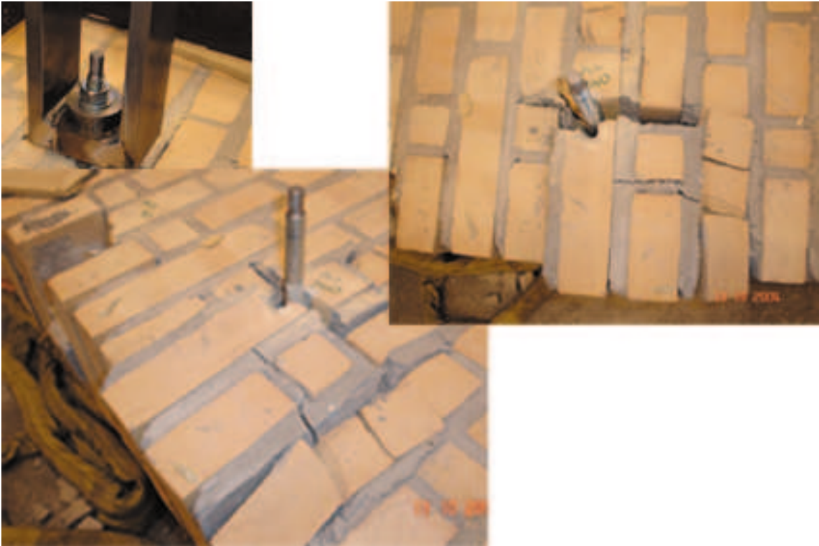
Figure A.135: The failure mode observed
