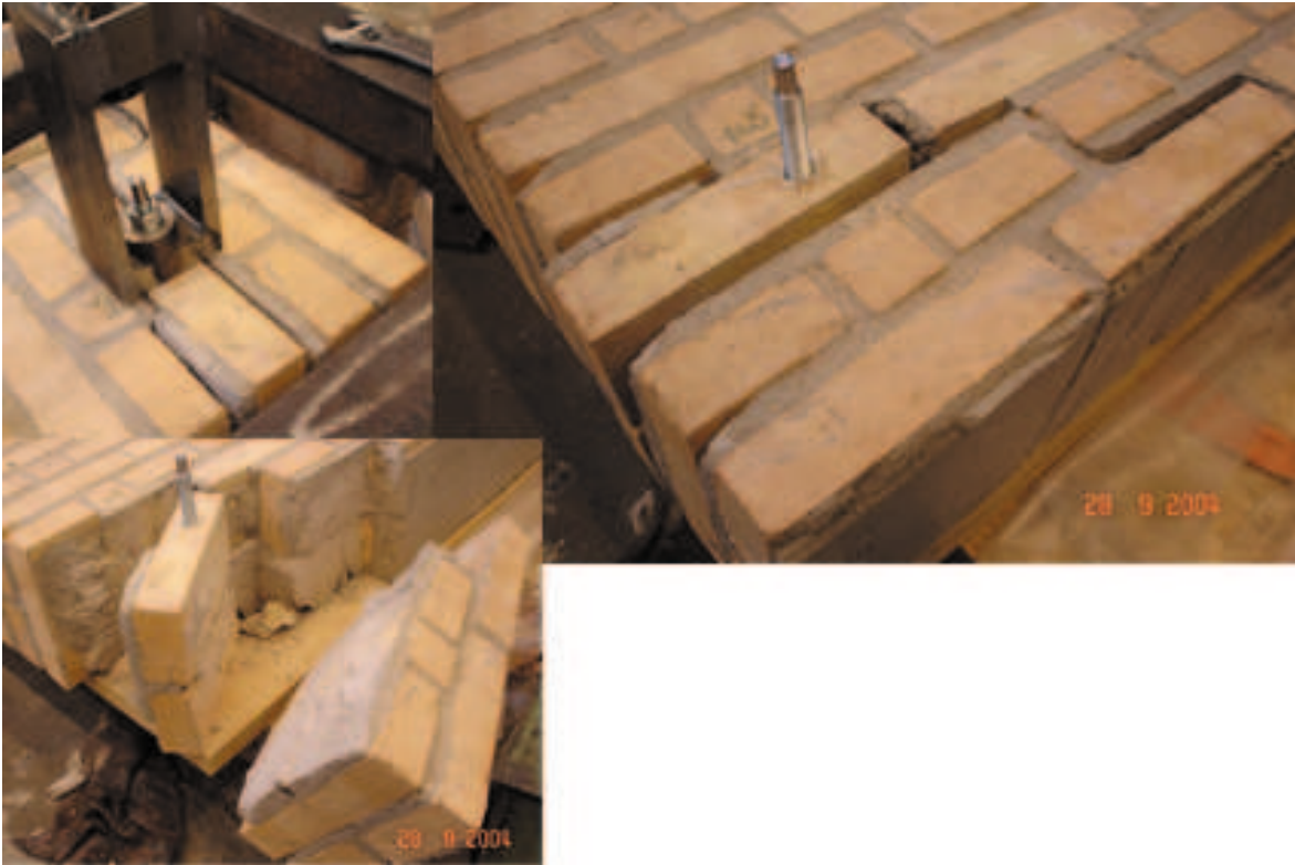
Figure A.119: The failure mode observed
