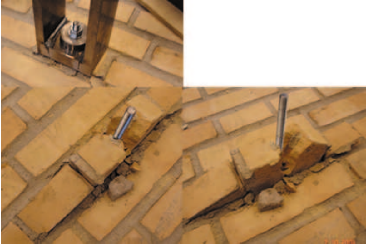
Figure A.43: The failure mode observed
