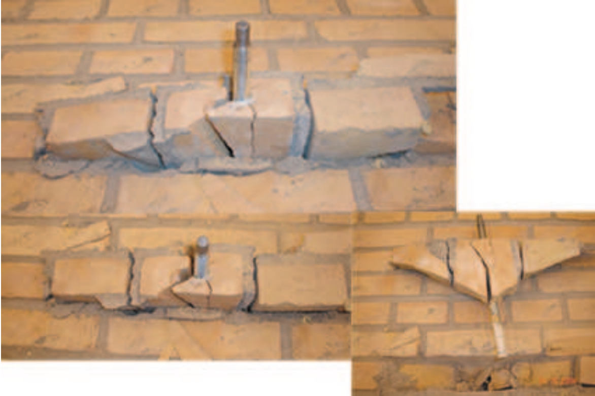
Figure A.49: The failure mode observed
