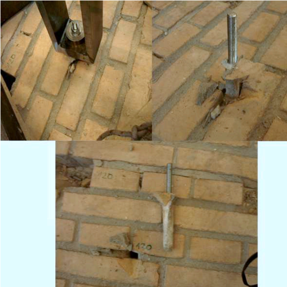
Figure A.95: The failure mode observed
