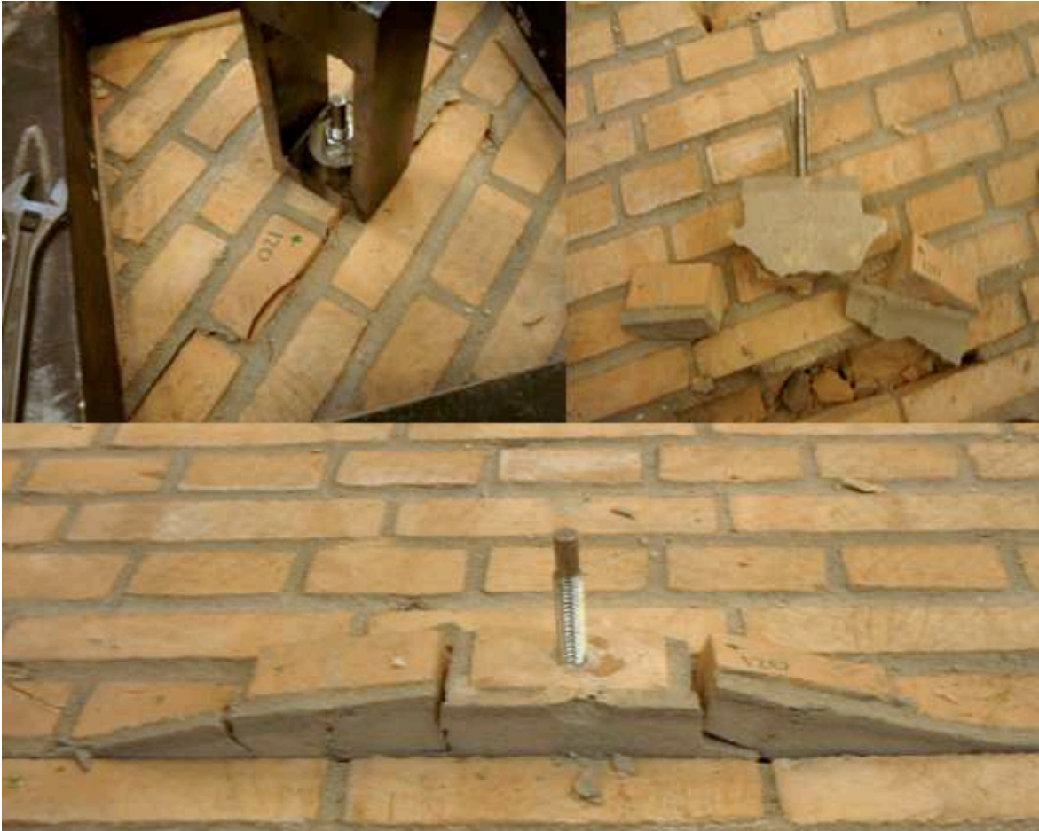
Figure A.79: The failure mode observed
