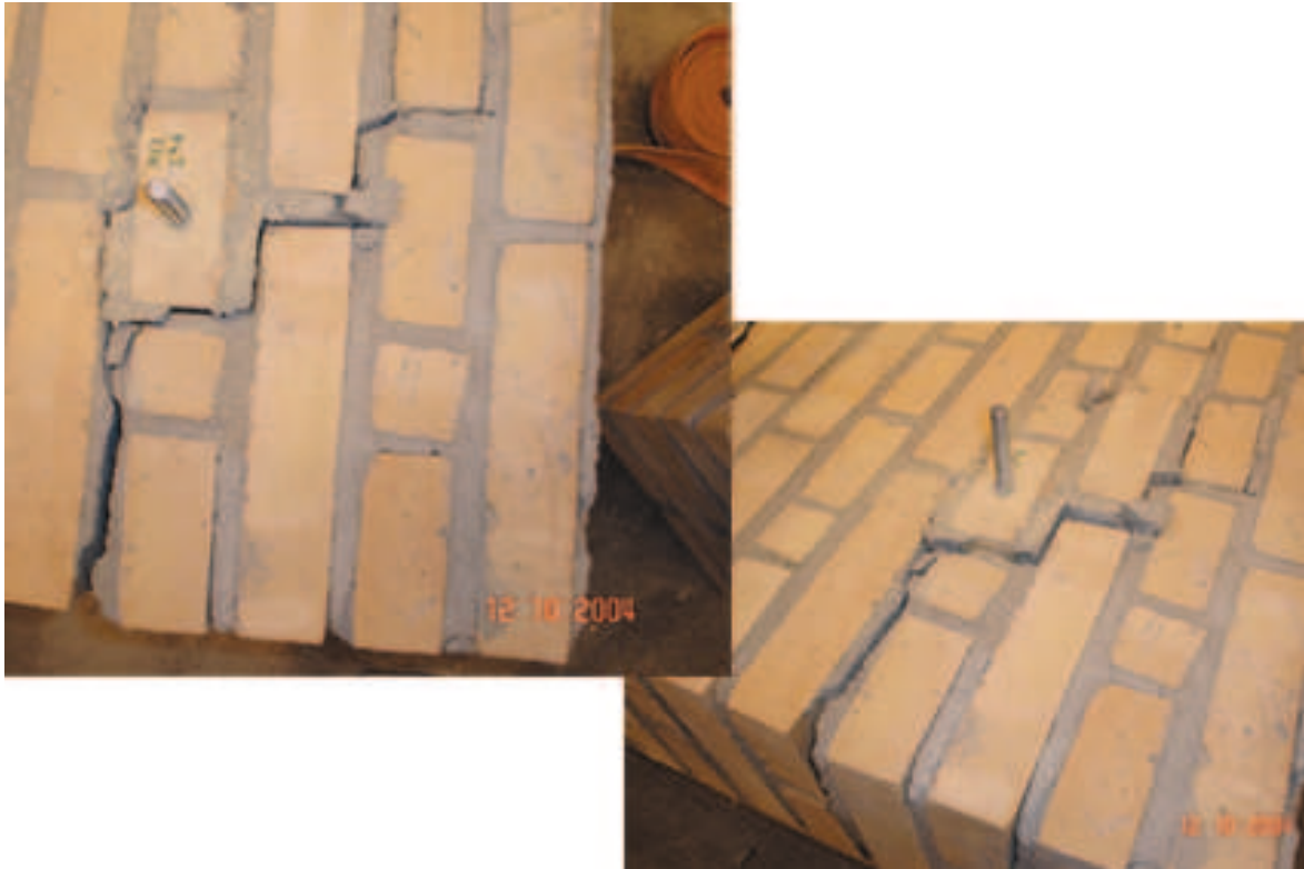
Figure A.115: The failure mode observed
