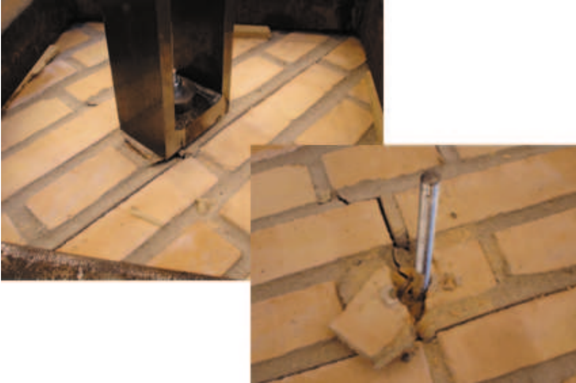
Figure A.41: The failure mode observed
