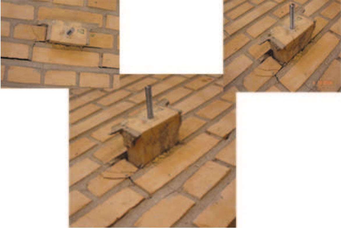
Figure A.143: The failure mode observed
