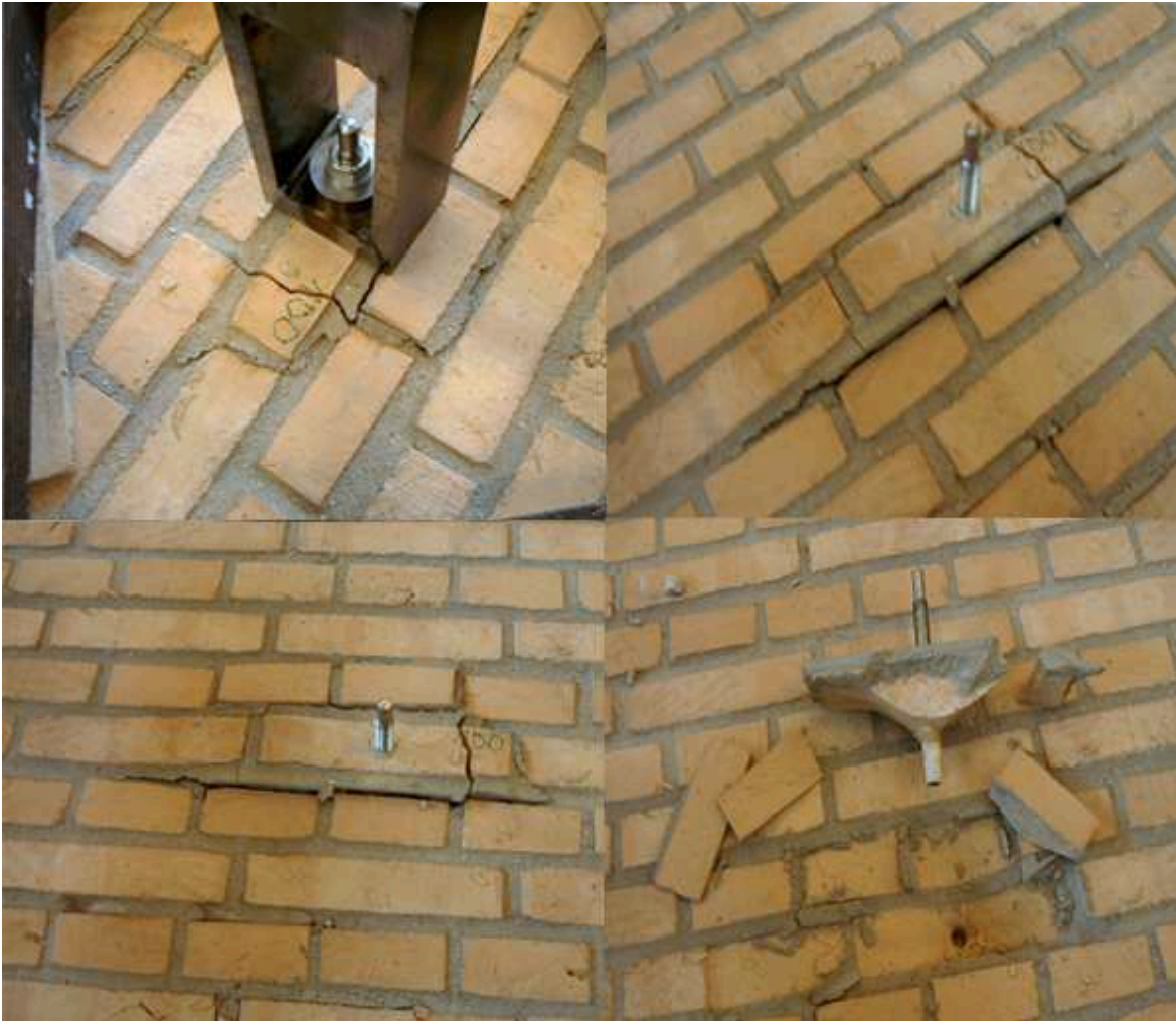
Figure A.31: The failure mode observed
