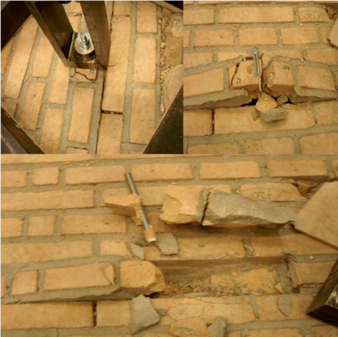
Figure A.69: The failure mode observed
