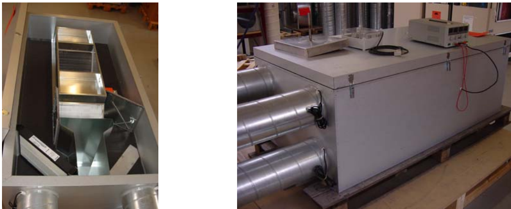
Figure 4 Pictures of the heat recovery unit.
