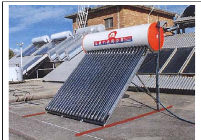
Figure 5. Water-in-glass solar water heater.
