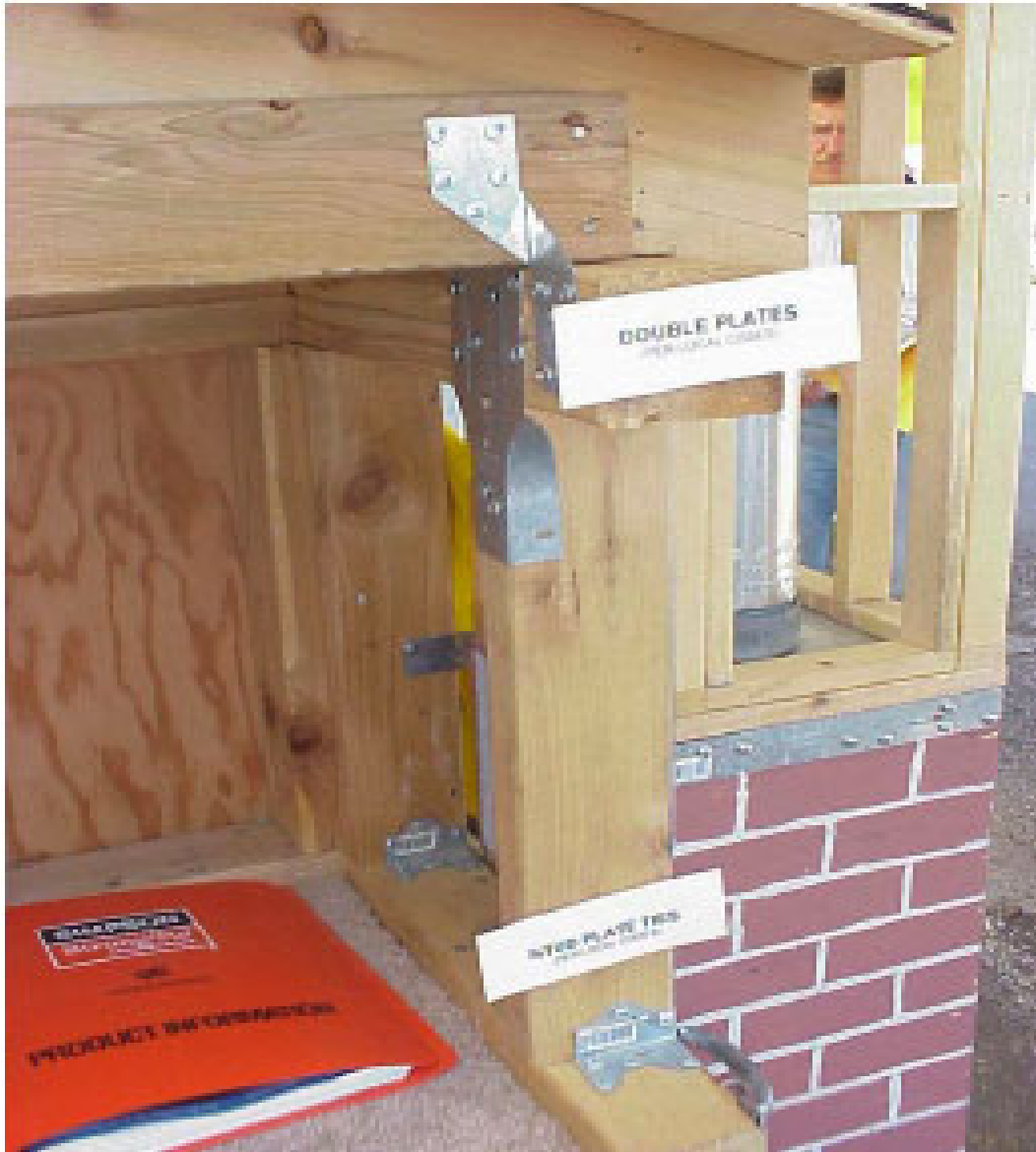
Figure 3: A model of various wall and roof joints showing seismic and wind anchors, which are commercially available and exceedingly worthy features in wind-prone and seismically active areas. The Alaska State Division of Emergency Services, motivated by the November 2002 earthquake, constructed this display. It is shown around the state as a public education display. (Photo by author).
