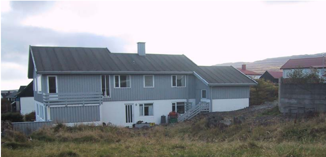
Figure 3 A typical Faroese single family house of a type that has been the dominating style since the 60'ies with full basement made of cement and the main living floor made of wood. It is common to expand the living area to the basement when the children want more space and privacy.
