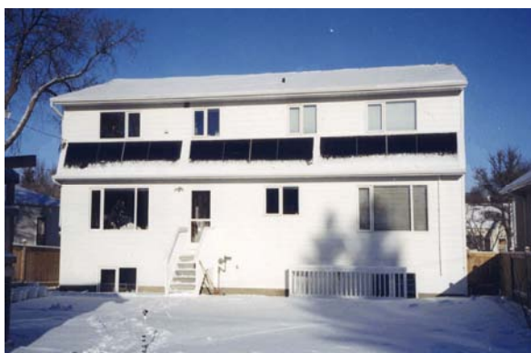
Figure 3. South side of the Dumont Residence, Saskatoon, December photo
