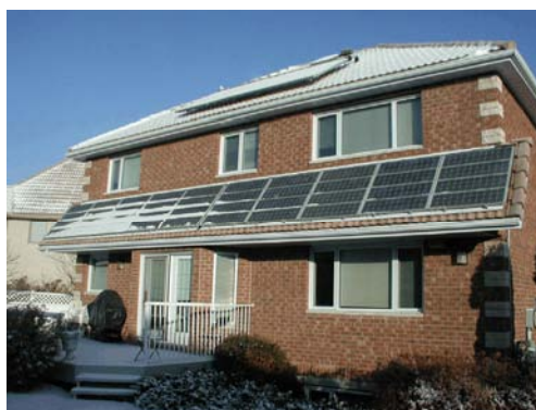
Figure 2. South side of the Saskatchewan Advanced House. One of 10 Advanced Houses built in Canada as part of a national project. Note the vacuum tube solar panels on the roof and the photovoltaic panels on the south wall. In very cold weather the snow will not readily melt off sloped surfaces.
