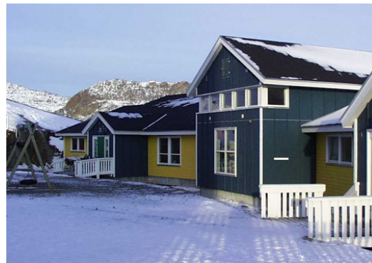
Kindergarten in Sisimiut
