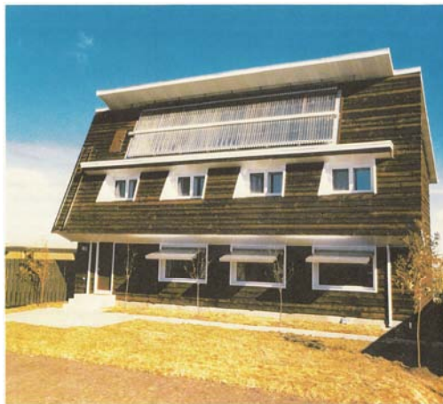
Figure 1. South Side of the Saskatchewan Conservation House, 1977. Note the active solar panels (vacuum tube) on the upper part of the south wall, and the insulating shutters on the lower windows. An 11,000 litre water storage tank was incorporated to store solar heat within the house.
