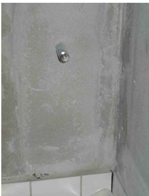
Billede 1 – Indmuret gulvregulator.
