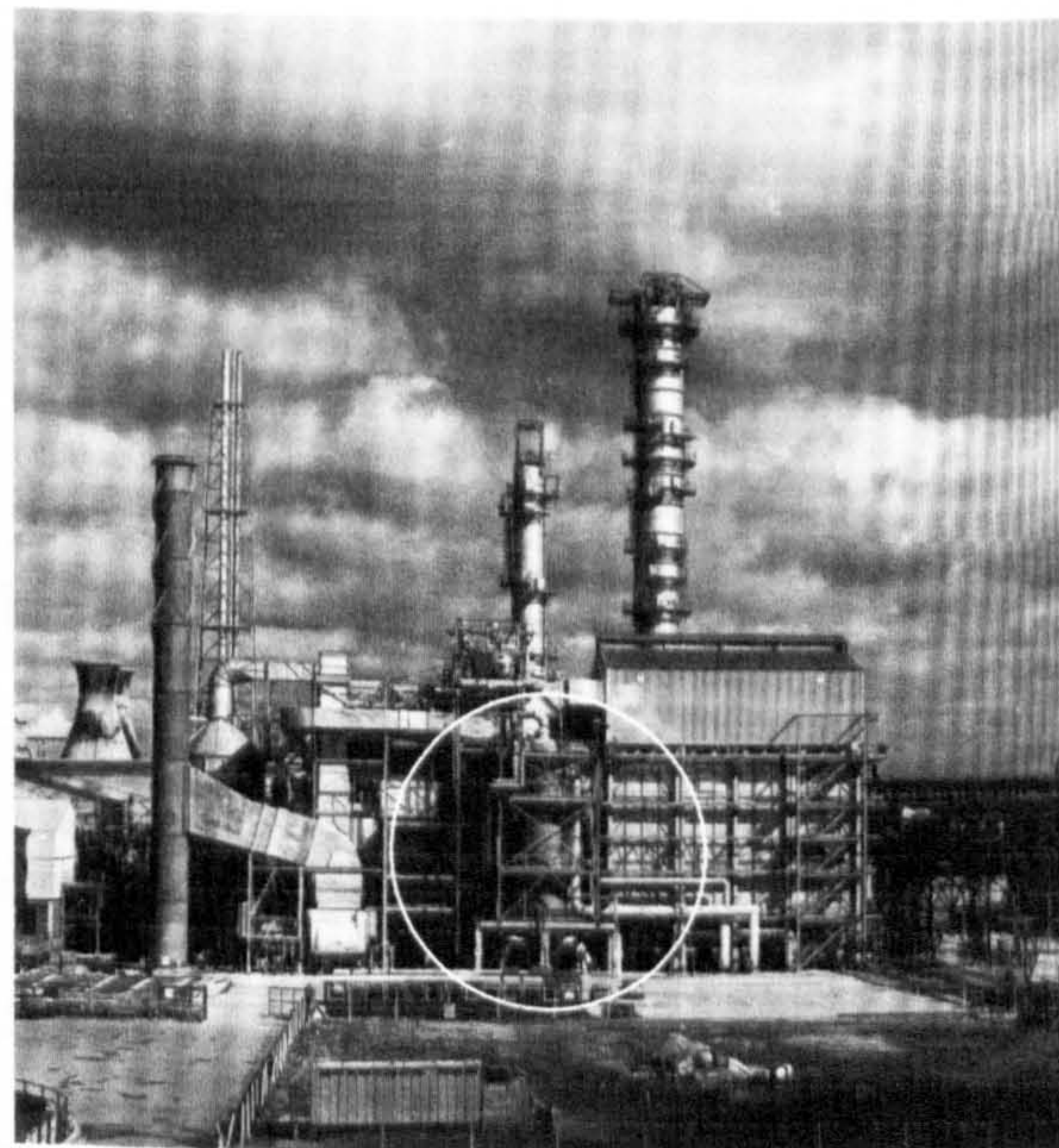
Figure 3.5.2.4: The top-fired reformer on ICI's No.4 ammonia plant at Billingham
