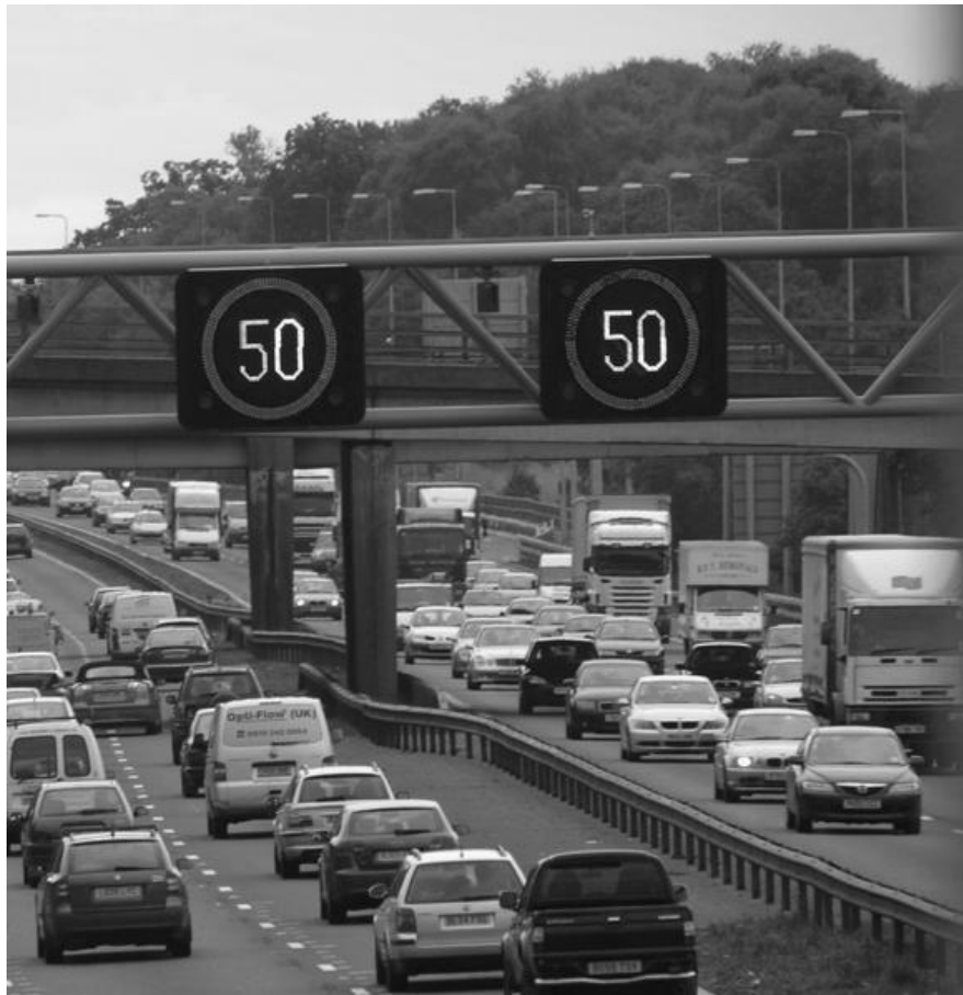
Figure 2.5: An example of variable speed limits sign setup on a highway [185].
