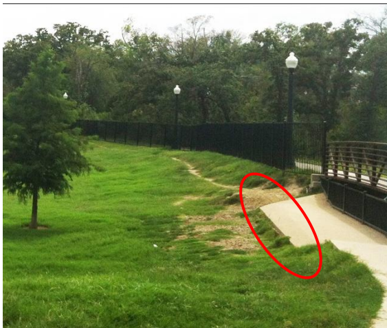
Figure 13: JPEG Image: Concrete "bench"
