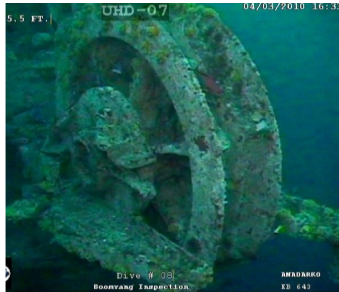
Fig. 3.5 Picture of mooring fairlead under the seawater.
