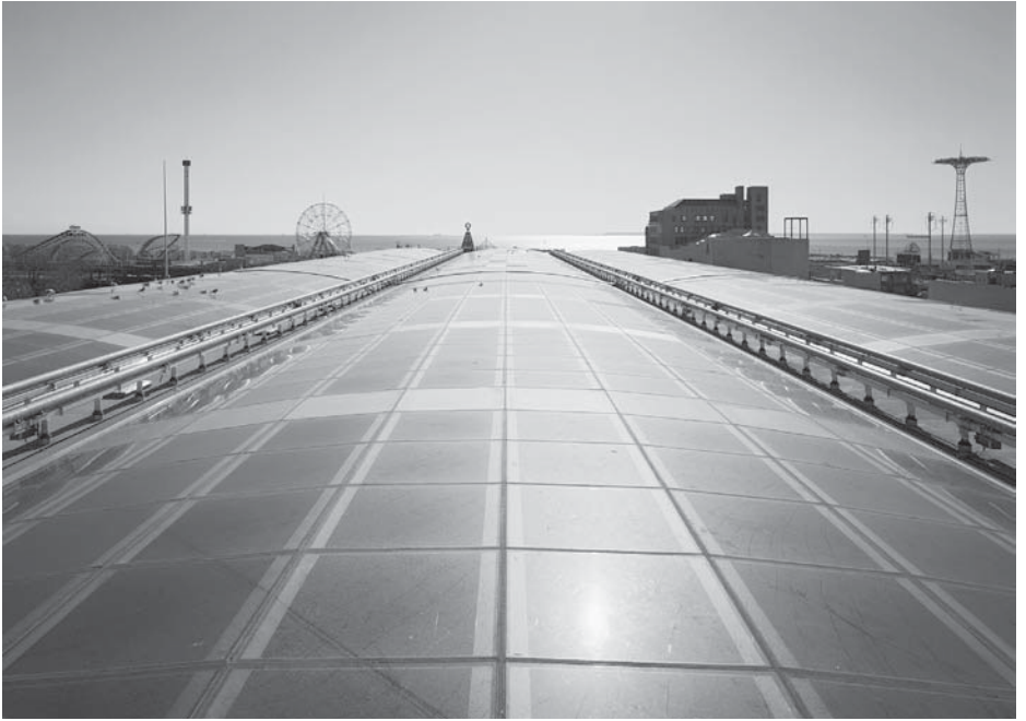
Figure 3 (Top) Exterior and (bottom) interior of photovoltaic glass enclosure above Stillwell Avenue subway station, Coney Island, New York.
