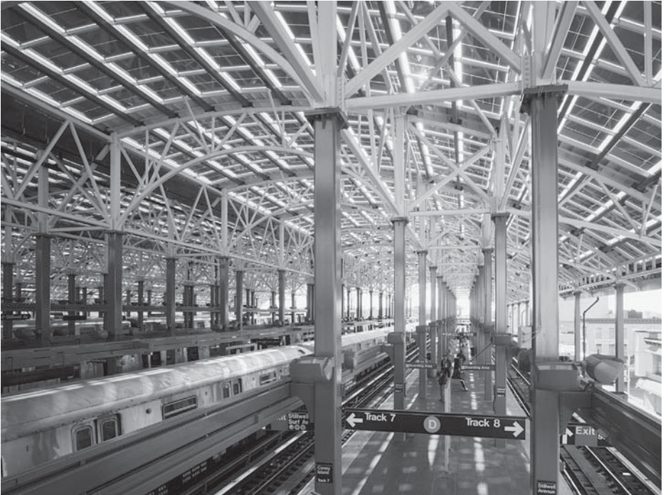
Figure 3 (Top) Exterior and (bottom) interior of photovoltaic glass enclosure above Stillwell Avenue subway station, Coney Island, New York.
