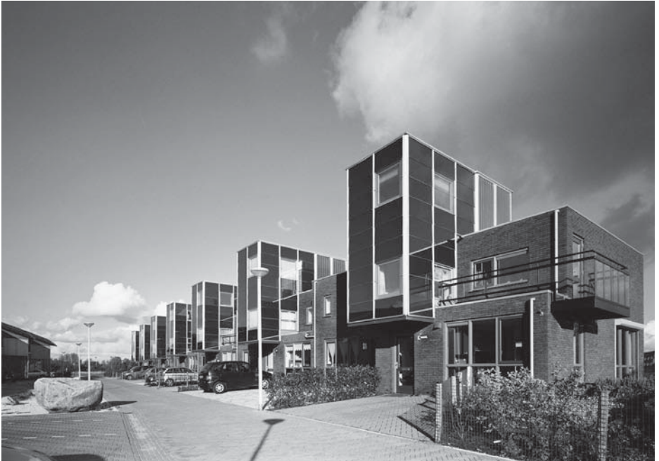
Figure 2 Intense green: Issselstein townhouses (built 2002).
