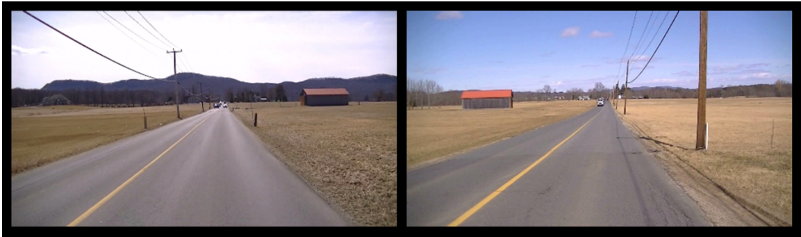
Figure 12 Static evaluation scenario with directional utility pole presence.
