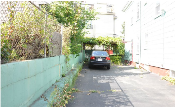
The large number of Impermeable front yards increase the surface runoff and non-point source pollution of the city.
