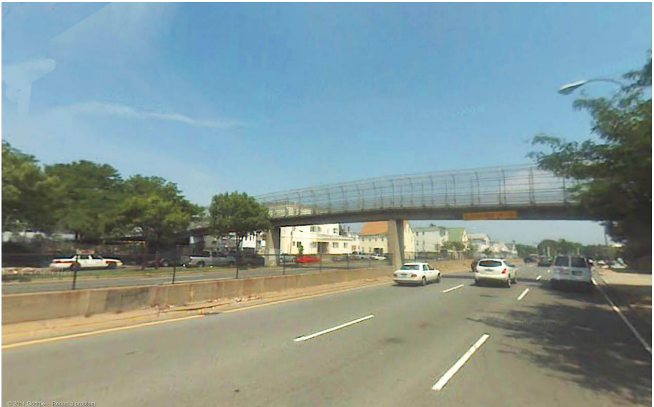
© 2011 Google Report a problem Otis Street Bridge before: A narrow pedestrian bridge crosses a sea of asphalt and 9 lanes of traffic, with no shelter from the elements.
