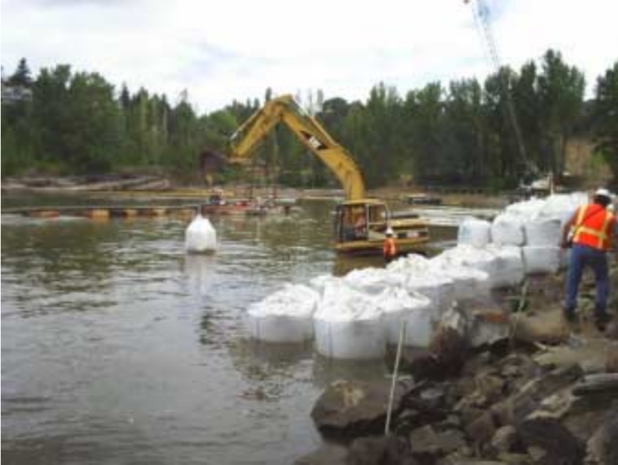
Figure 1. Deployment of Organoclay Cap at Willamette River
