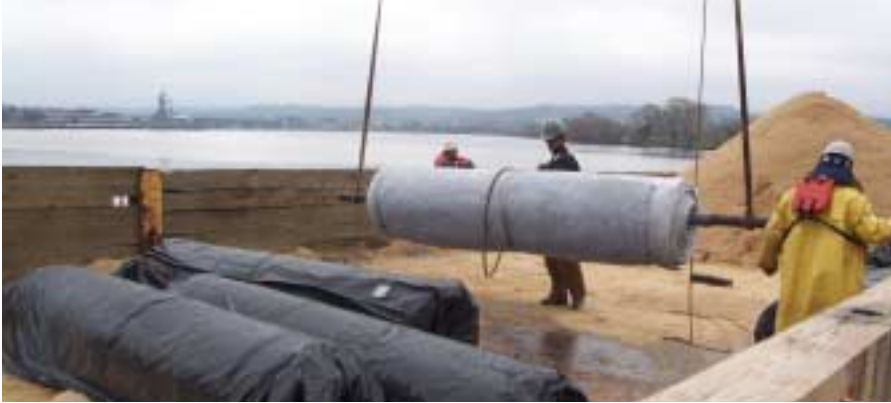
Figure 3. Reactive material mat being prepared for deployment on the Anacostia River
