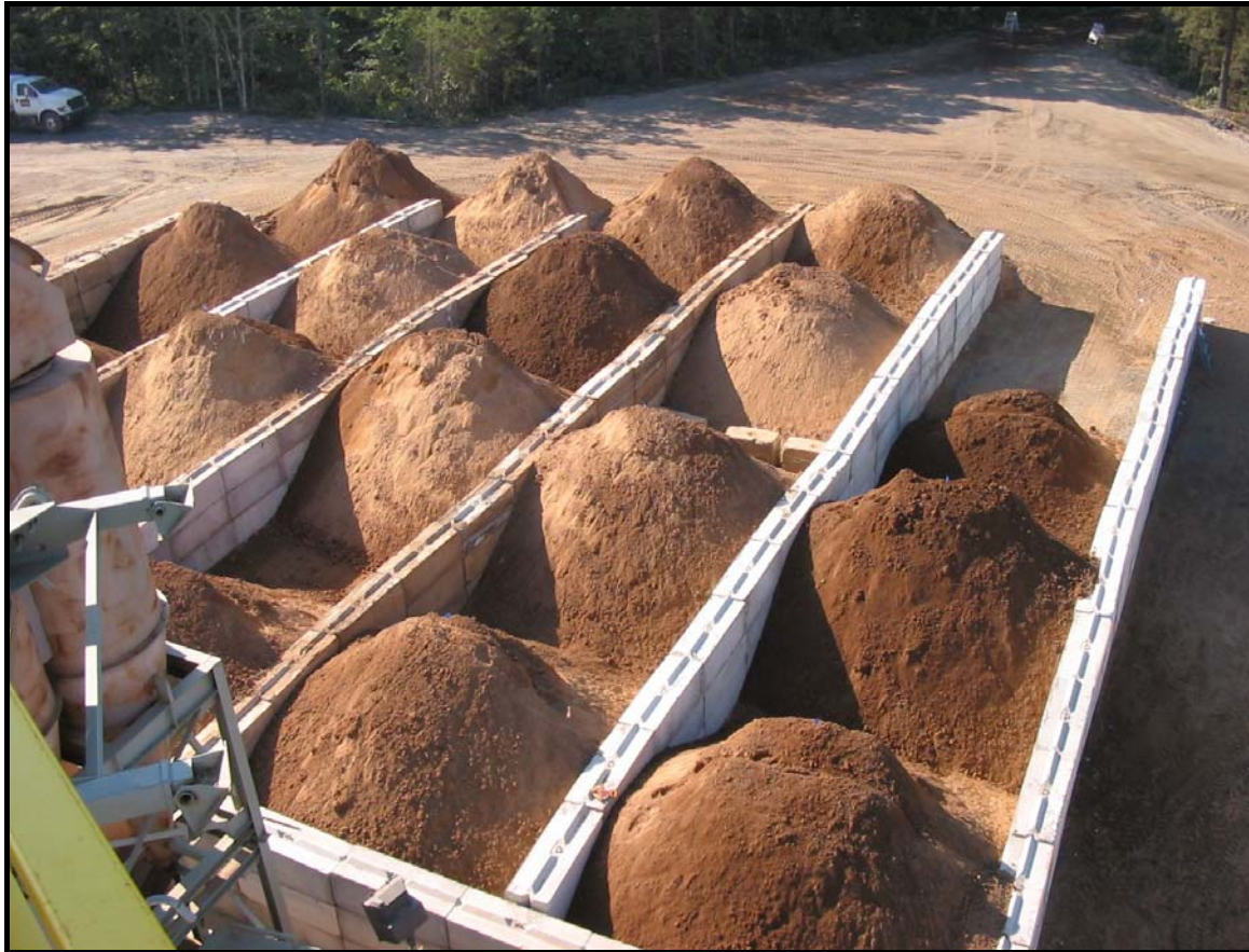
Figure 7. Site Infra-structure re-designed for 100 cy piles
