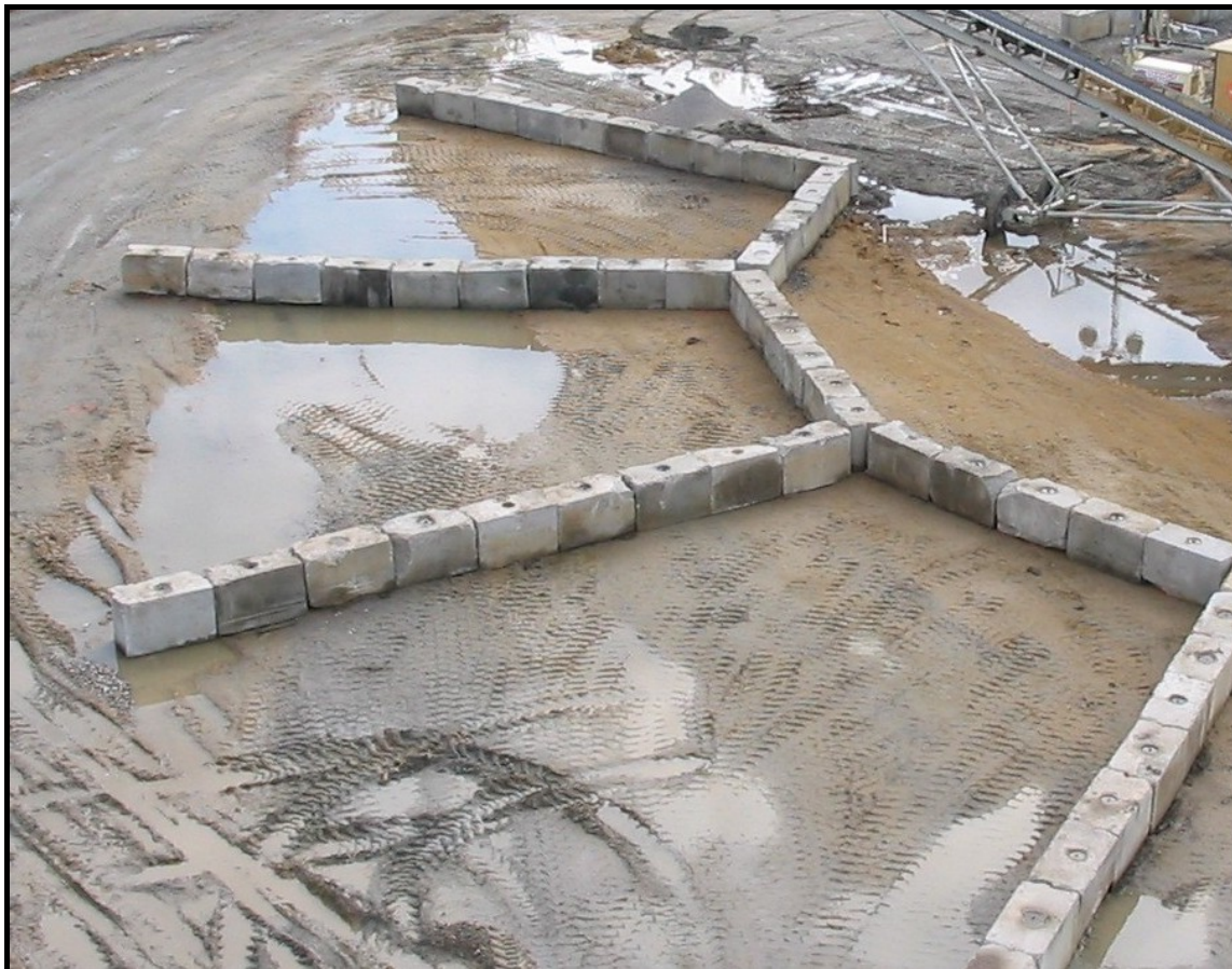
Figure 6. Site Infra-structure designed for 500 cy piles
