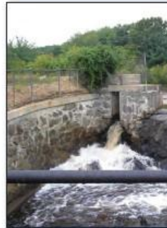
Figure 1. Maxwell Pond Dam on Black Brook in September 2008.
