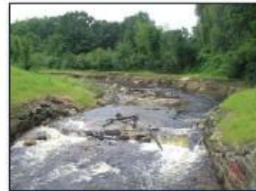
Figure 2. Same location as Figure 1, showing Black Brook in June 2009 after the dam was removed and natural gas line relocated.
