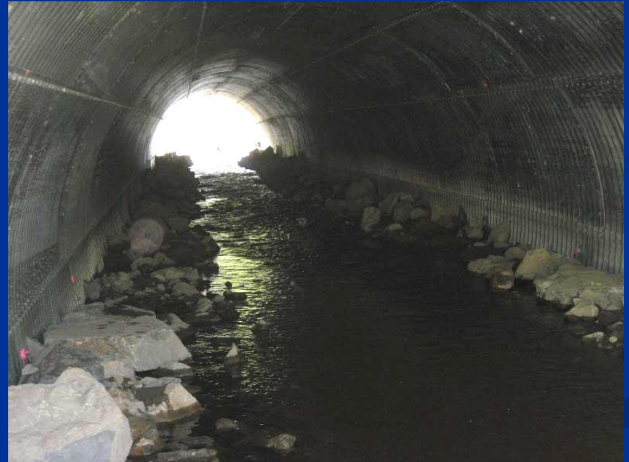
Coal Creek, Kenai (12 foot channel in 18 foot pipe)
