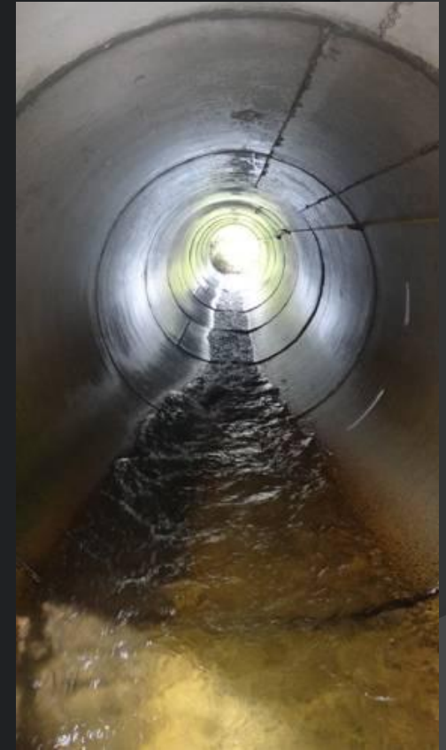
Smooth concrete culvert Elsa Goerig (INRS) 2011
