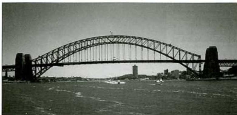
Harbor Bridge, Sydney
