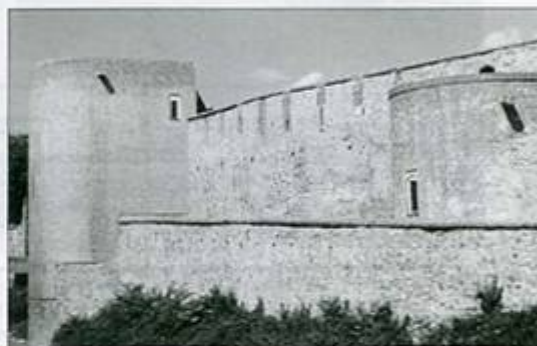
Old City Walls
