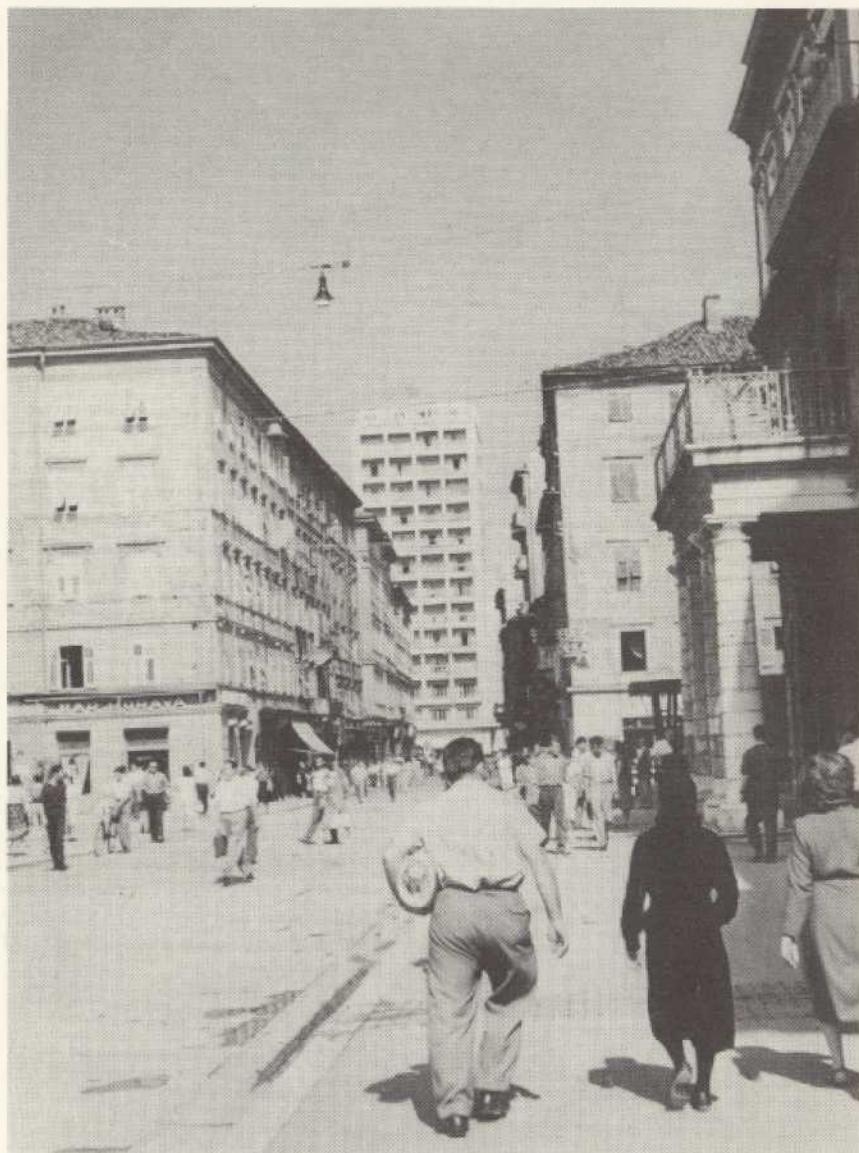
The harbor city of Rijeka, Yugoslavia's most important seaport, has recovered from severe war damage. In the background the tallest building is topped with a prominent red star.
