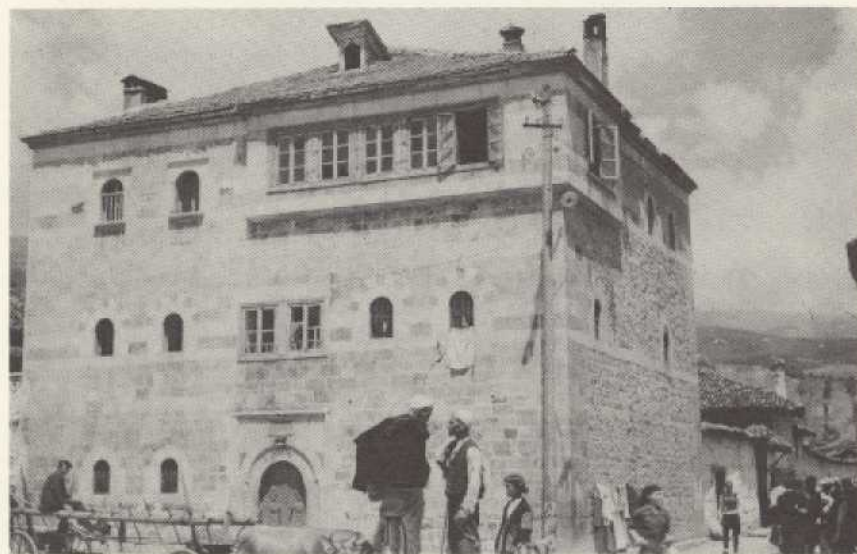
The streets of Peć are faced with tall poplars and with open drainage streams flowing along in shallow ditches. On the main street is this fine example of the thick-walled, fortress-like Albanian houses, with tiny windows and living quarters on the uppermost story.
