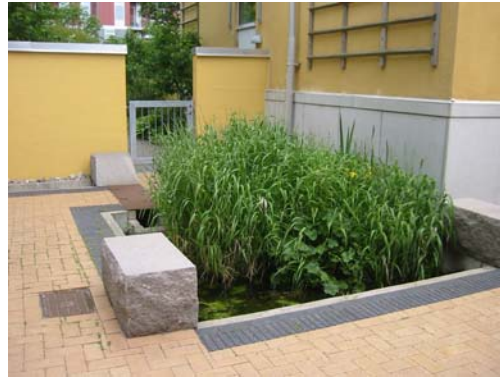
Figure 4. Stormwater Street Planter
