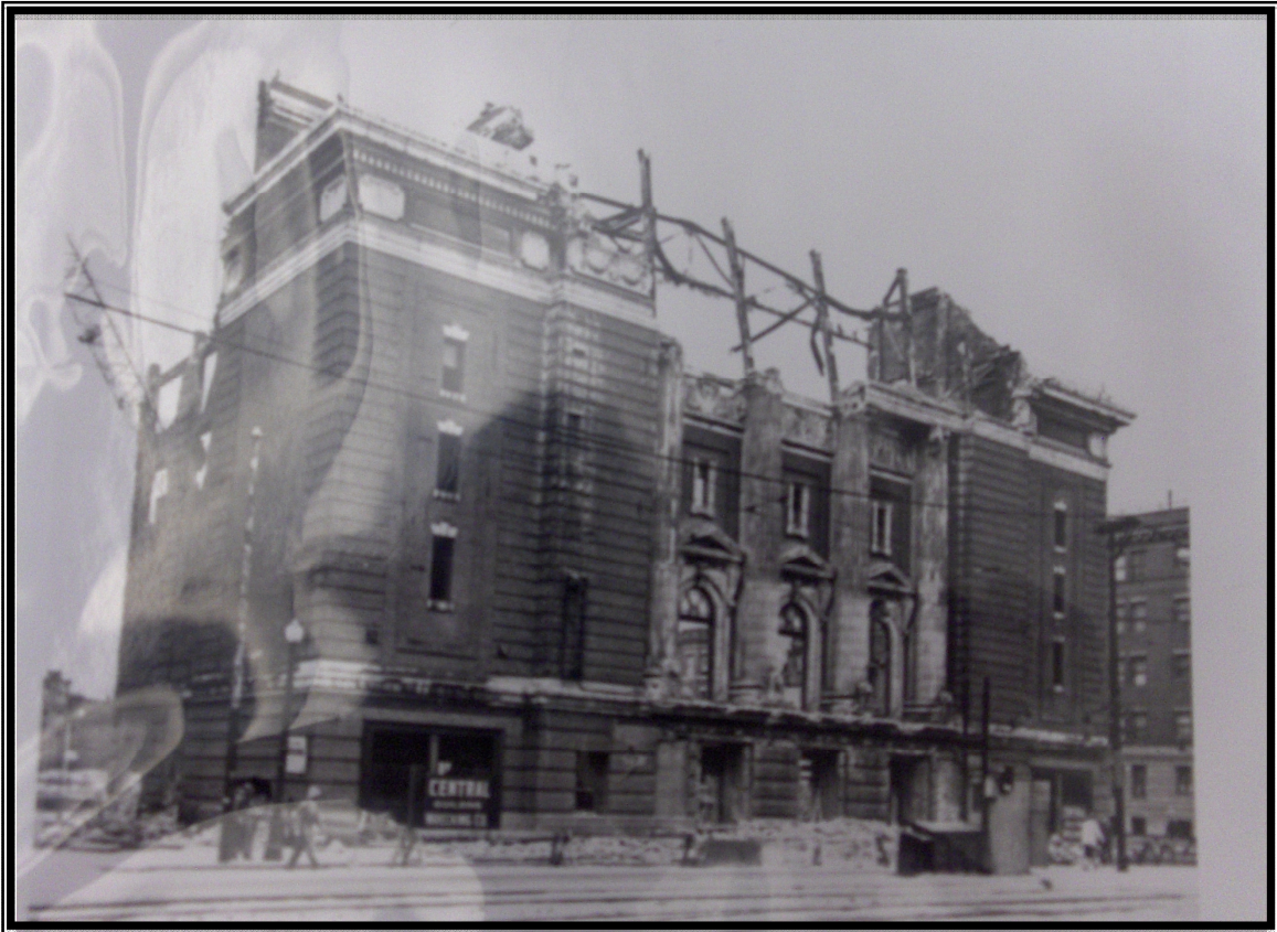
T. Boston Opera House during demolition.
