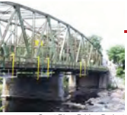
Great River Bridge Project
