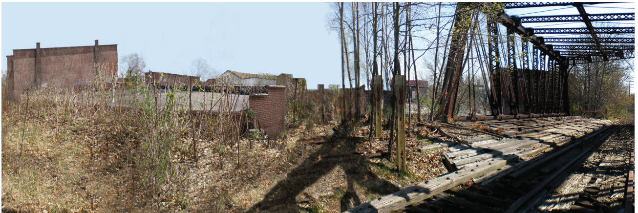
Existing view at Rail Trail at Elm St Bridge
