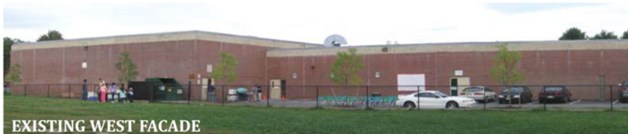
EXISTING WEST FACADE
