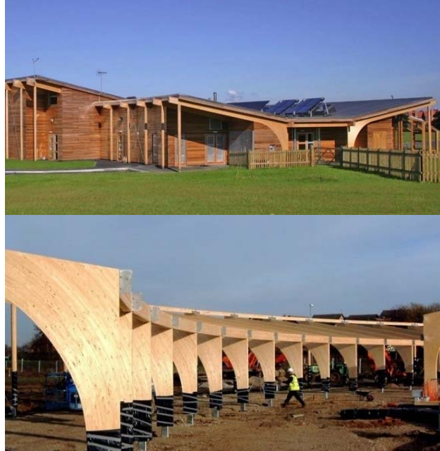
Figure 13 (Top to Bottom): Kingsmead Primary School, Glulamined Structure during construction (White Design).
