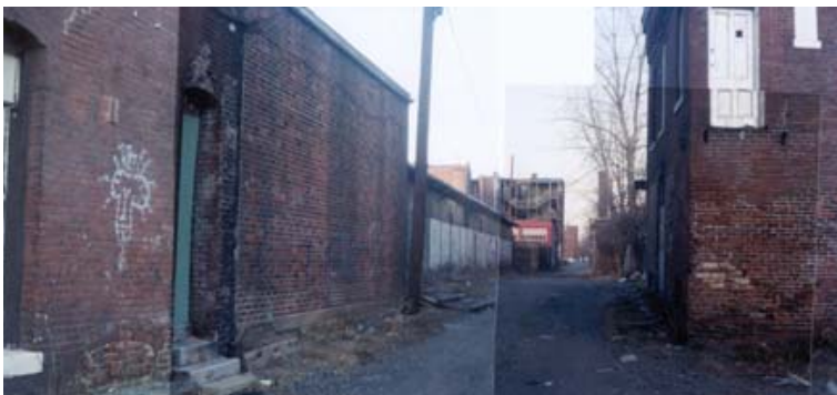
Figure 15: Alley between Main and Clemente Streets in Holyoke, Massachusetts. This poorly kept alley is filled with trash and graffiti.
