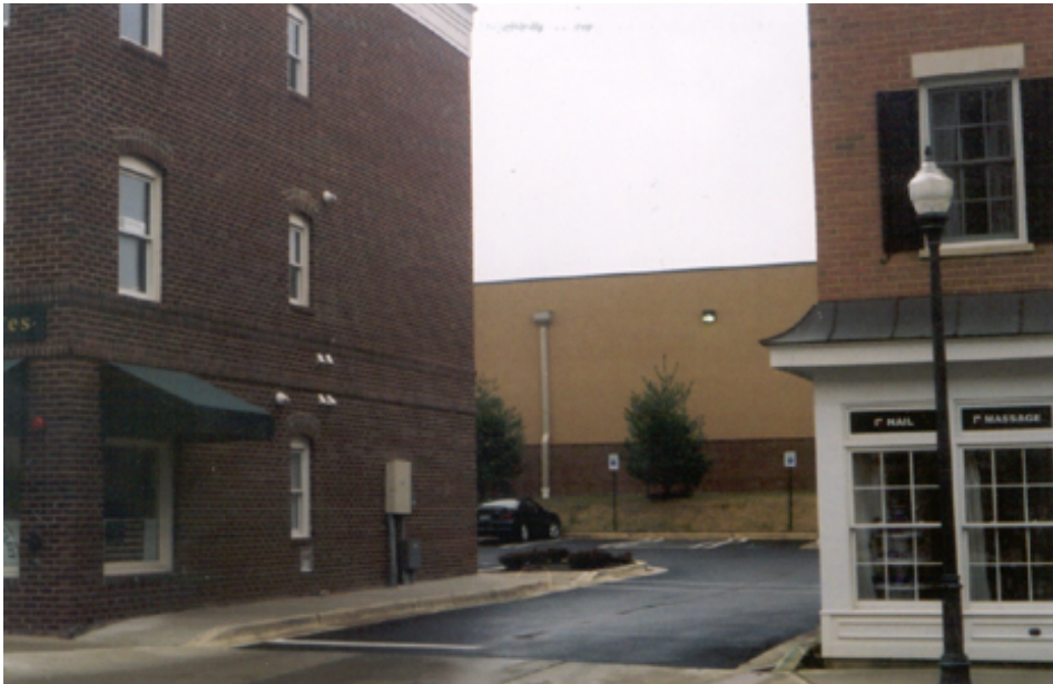
Figure 49: The alley connecting to the parking area is little more than a driveway with walls.
