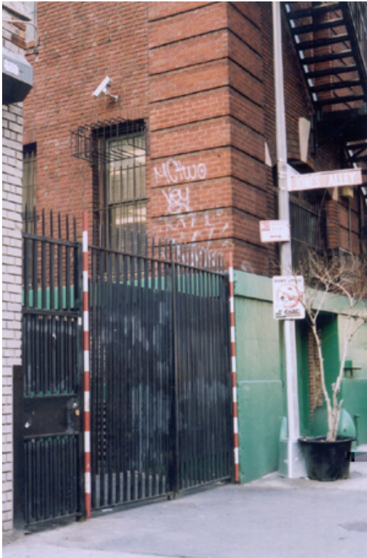
Figure 44: Gates limit access to Jones Alley.
