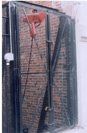
Figure 38: Dumb waiters move goods from the street to the alley's lower level.
