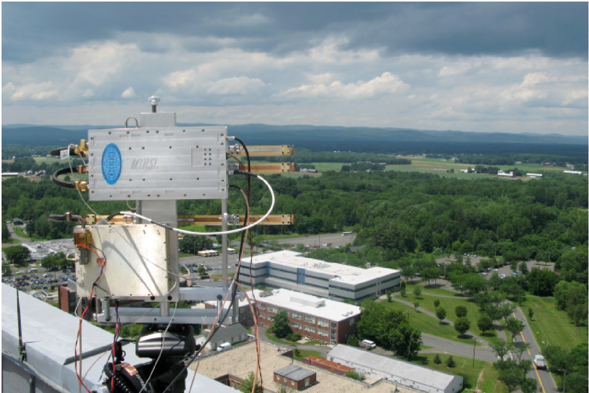
Figure 6.5. Picture of the UMass Ka-band interferometer deployed on the rooftop of the LGRT
